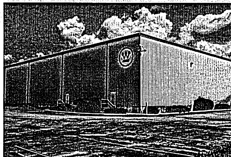
Photo 24: Northwest corner, facing southwest.
