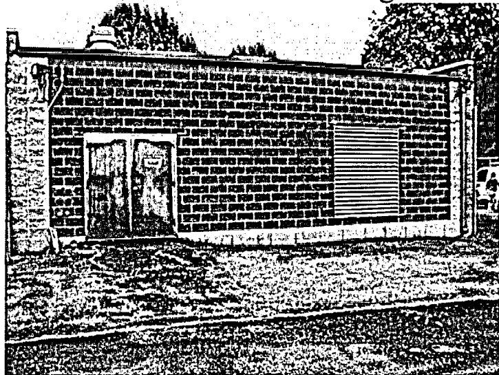
Photo 63: South wall, inside fence, facing north.
