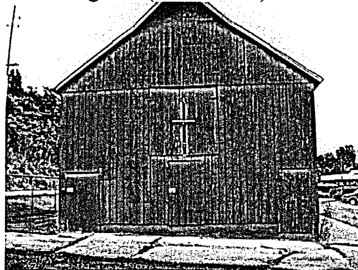
Photo 72: West wall facing east.
