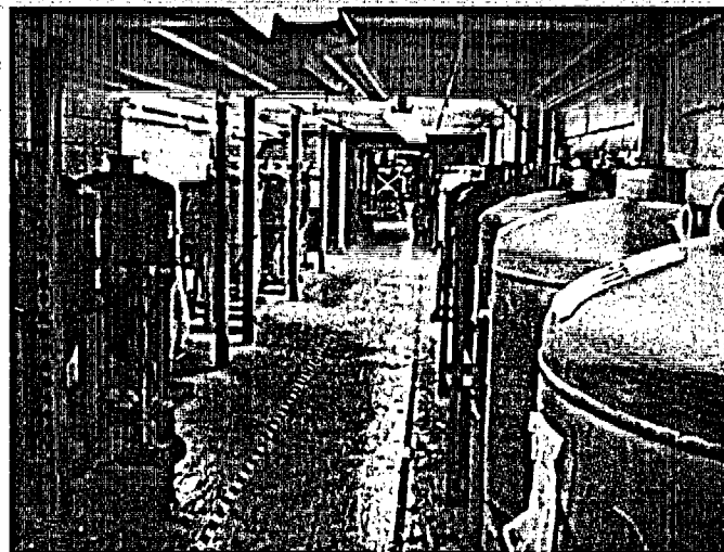
Photo. 139: BLD Hopper storage area, facing west.
