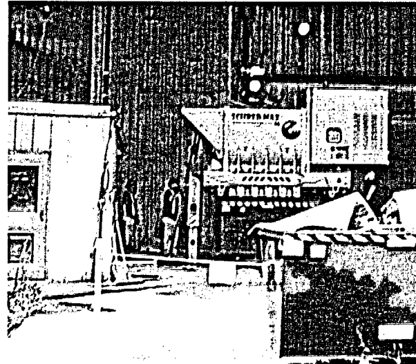
Photo 80: Shredder room, facing north.
