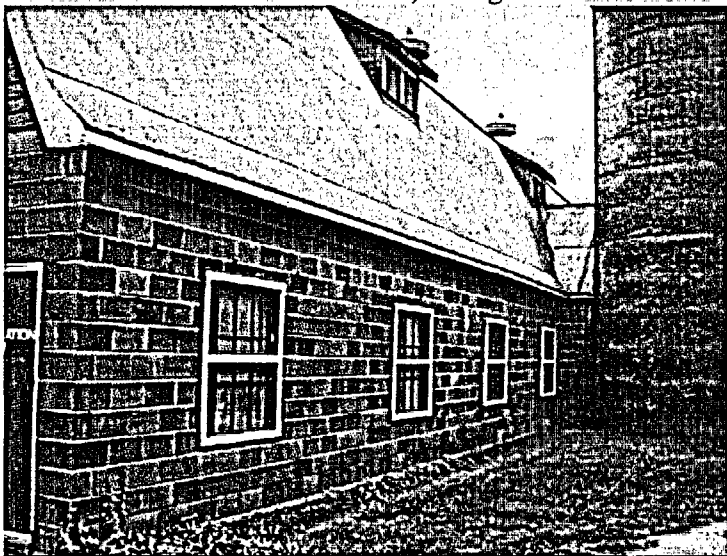
Photo 69: North wall, facing southwest
