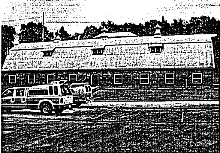
Photo 67: South wall, facing north.
