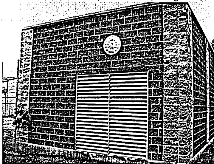
Photo 66: East wall, outside fence, facing west.
