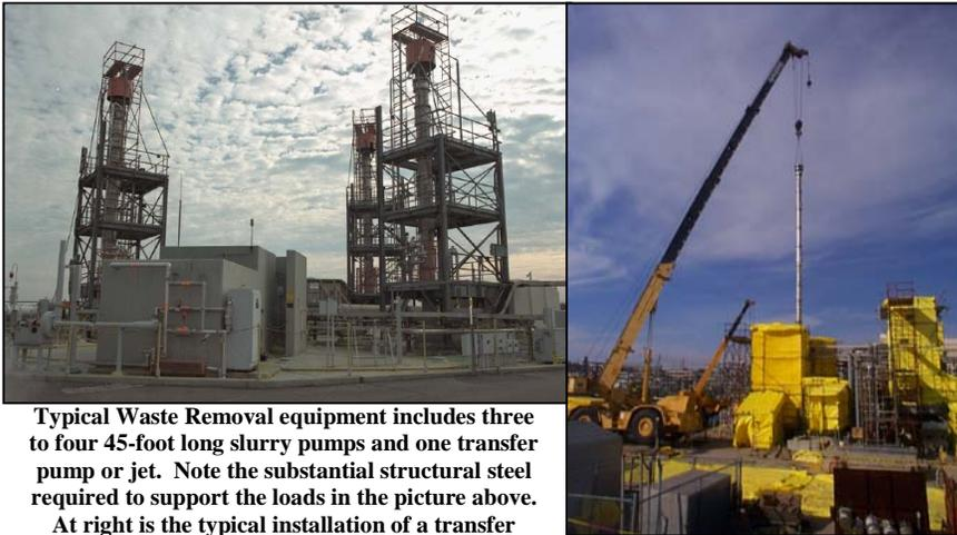
Typical Waste Removal equipment includes three to four 45-foot long slurry pumps and one transfer pump or jet. Note the substantial structural steel required to support the loads in the picture above.
