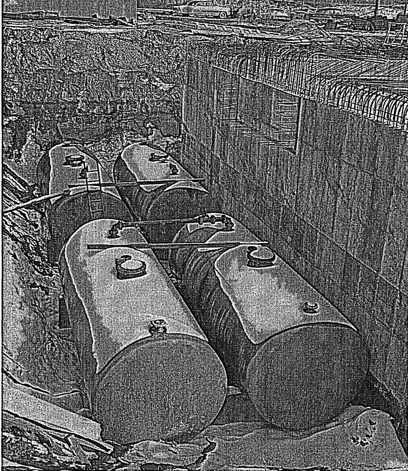
PHOTO 5. EXCAVATION WITH HRA TANKS IN PLACE ORIGINAL DATED 12 JAN 1959
