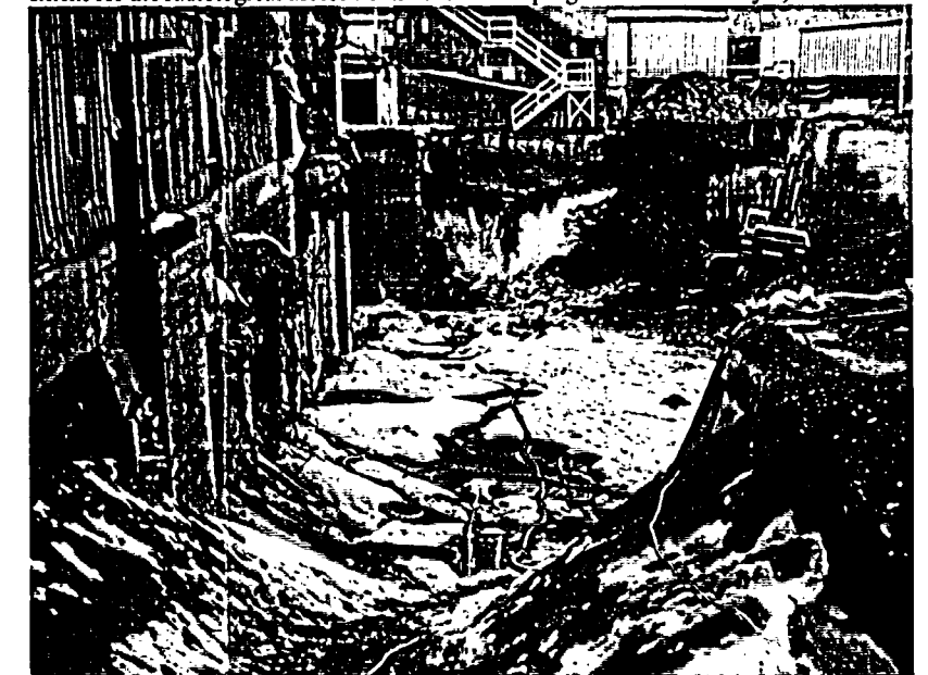
Picture 2 – Current view of the excavation facing south. The excavator, located in the footprint of the former Waste Disposal Building, delineates the approximate northern extent for the radiological assessment. Excavation progress as of February 7, 2005
