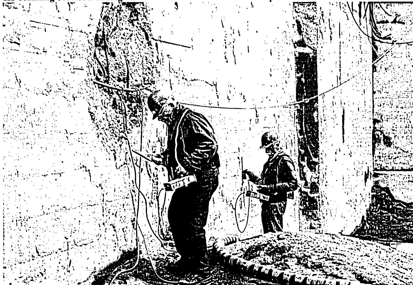
HP scanning Service Building wall with beta sensitive scintillation probes.
