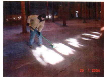
Photo 5-4. Floor preparation prior to static measurement collection.
