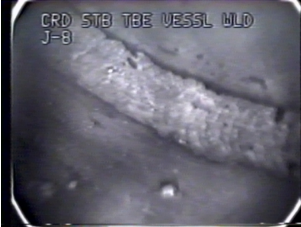
Figure A.7 Frame Capture from Videotaped Visual Inspection of a Control Rod Drive Stub Tube Weld. Note the relatively soft focus.
