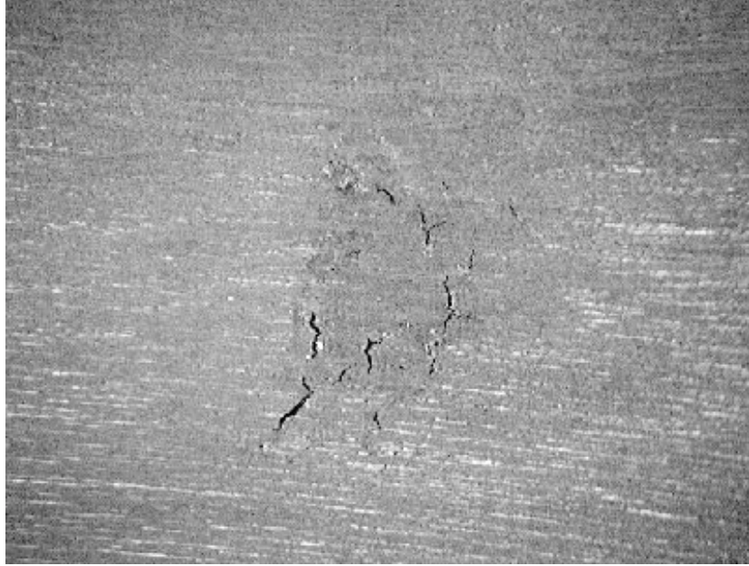
Figure 4.1 Cracking in Reactor Pressure Vessel Cladding as Imaged by a DIAKONT Closed Circuit Video System (Vasiliev et al. 1999)
