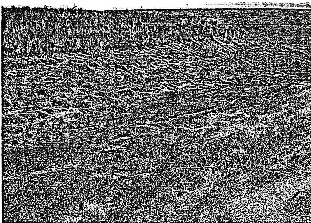
Damp area in roadway between ponds #3 & #4. Damp area was in line with wheel way of vehicle traffic. Date: 10/19/04
