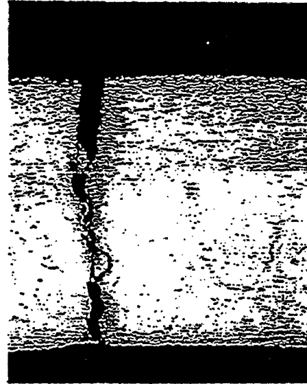
Figure 5c: The fissure of fig. 5b becomes a penetrating crack at level 395 bfc.
