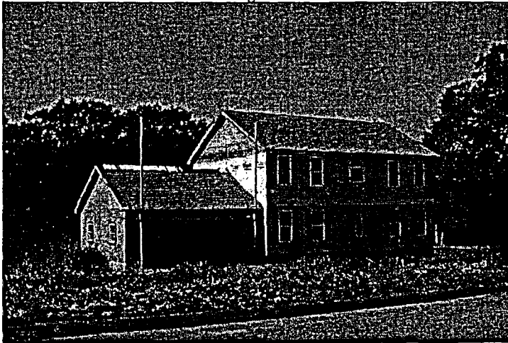
New Housing Construction
