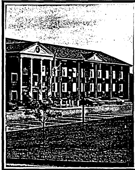
Elderly Housing AHEPA on Clark Lane
