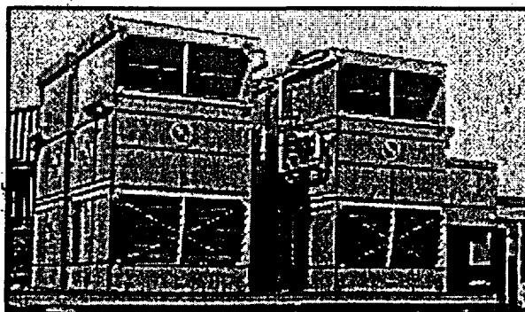
HXV installation with optional flow control package for comfort cooling application.
