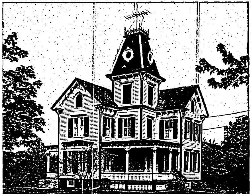
Mid-century French Second Empire style is represented by this "outstanding" 189 Great Neck Road house. Bracketed eaves, mansard-roofed tower with empty "clock face" windows and the gingerbread-decked verandas identify the period.
