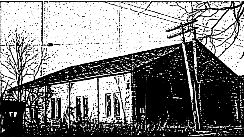
This three-bay concrete-block car barn facing the Niantic River Road was next to the power substation that housed two 300KW rotary converters. Initially supplied by the New London Gas & Electric Co. with a 4,600-volt line, in 1911 an 11,000-volt high transmission line from the Shore Line Electric Railway's Saybrook power station supplied the power for the converters.
