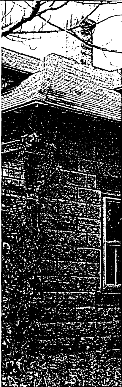
A cut-granite foundation supported the elaborate concrete block 1905 "workman's temple" at 436 Boston Post Road. Values then featured new man-made material, while burying the very traditional one it copied. Henry Beebe (listed as a mason in the 1900 census) owned the land. With the details of a mansion, beaded mortar joints separated the numerous molds of man-made blocks. Quoins, sills and lintels were of brownstone color in contrast with the granite-colored body of this masonry masterpiece. Opposite: Millstone quarry in 1966, just days before it was bulldozed. The former quarry was opened to the Sound to become an environmentally friendly substitute for the huge cooling towers otherwise required.
