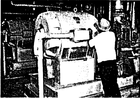
BOILER FEED PUMP MOTOR #4-3
