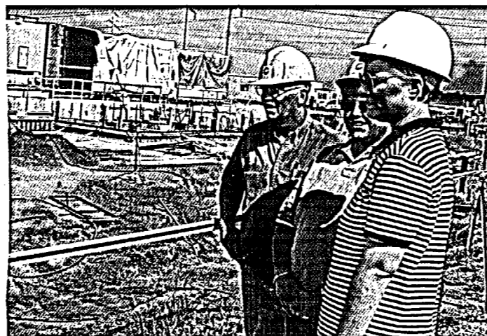
Employees tour the Wisdom Unit 2 construction site.
