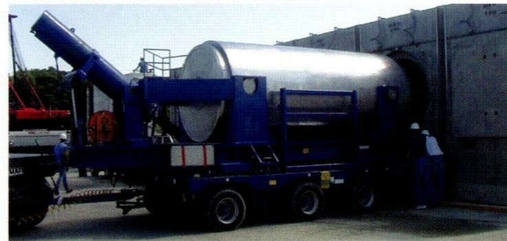
Canisters filled with used nuclear fuel are moved into on-site dry-storage facilities at the Duane Arnold Energy Center near Palo, Iowa.
