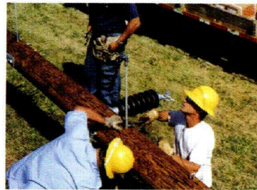
Linemen frame a transmission pole for the Willemssen-Blairsburg line.
