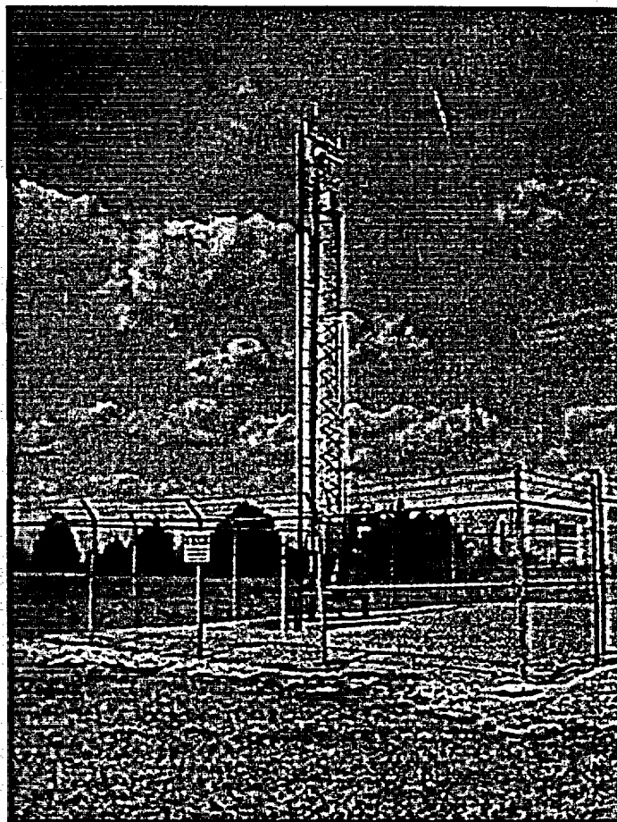
Pictured is the Secondary Meteorological Tower. This station obtains measurements at a height of 10 meters, and provides backup data for the Primary Meteorological Tower readings at 10, 60 and 90 meters.
