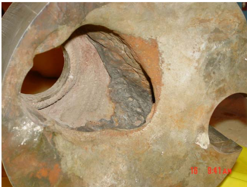
Figure 7. A photograph of the 18-inch diameter section of the discarded Davis-Besse head, containing the corrosion cavity created by leakage from the included nozzle (#3).
