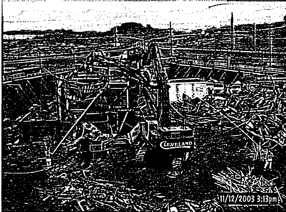
Photo 5 - Demolition of secondary crusher
