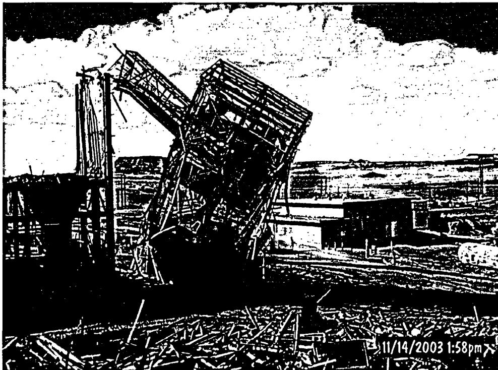
Photo 6 - Demolition of Sample Tower
