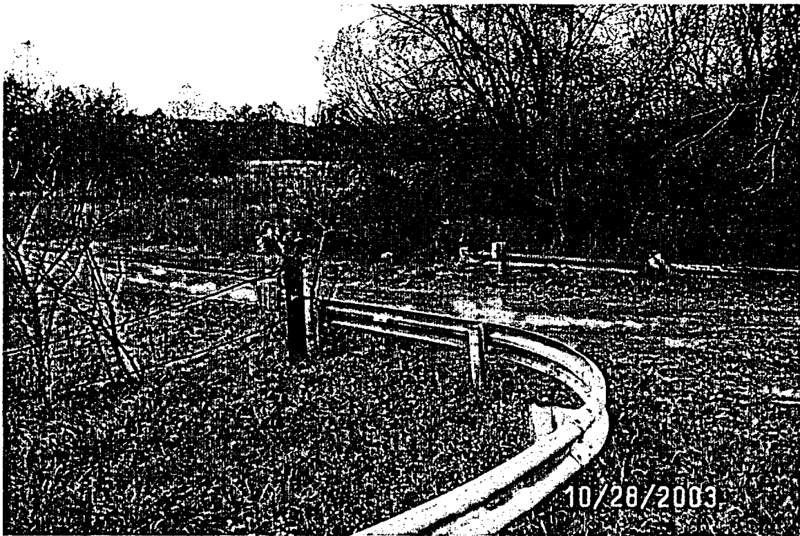
BUR 10/2003. PL-1. Location of the former access gate at Strangford Road.
