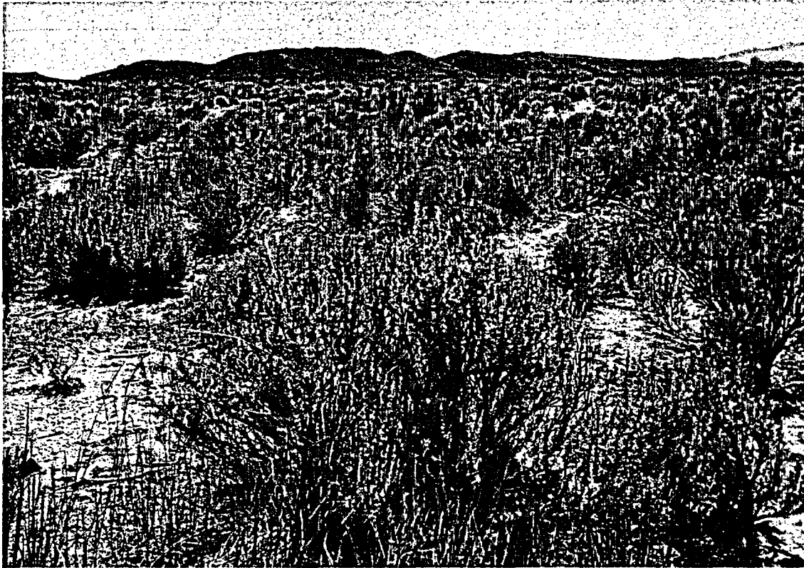
LKV 6/2003. PL-1. Shrubs growing on the top slope of the disposal cell.
