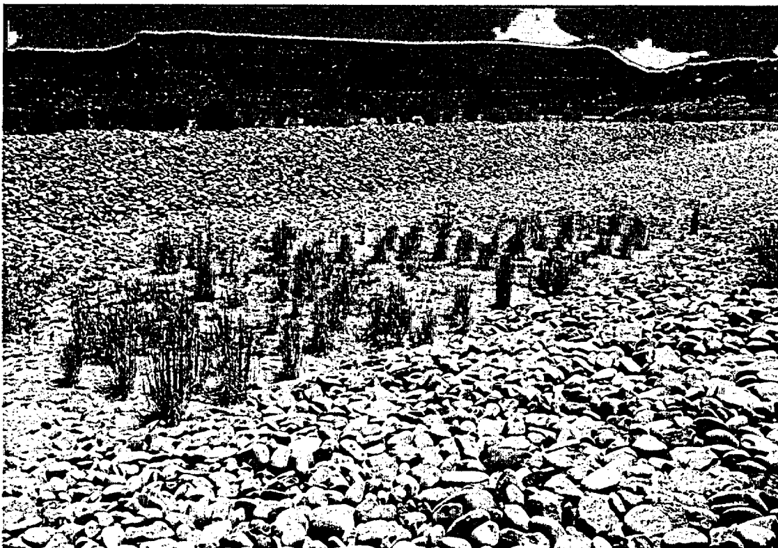
NAT 07/2003. PL-2. Sediment accumulation in the interceptor channel.
