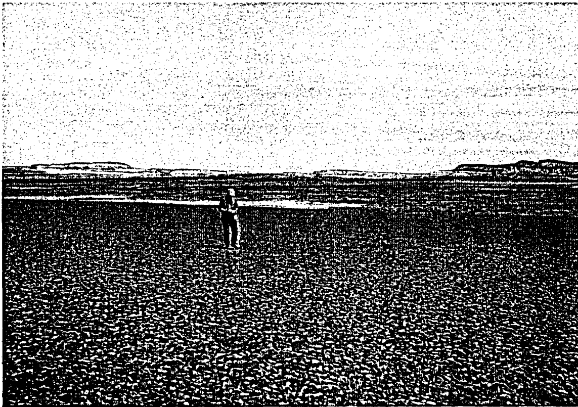
AMB 5/2003. PL-3. Circular-shaped vehicular disturbance on the north facet of the cell cover.
