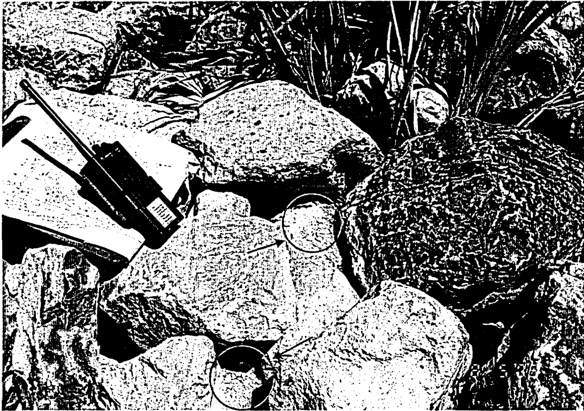
MAY 8/2003. PL-3. Evaporite deposits on apron riprap at the east corner of the cell.
