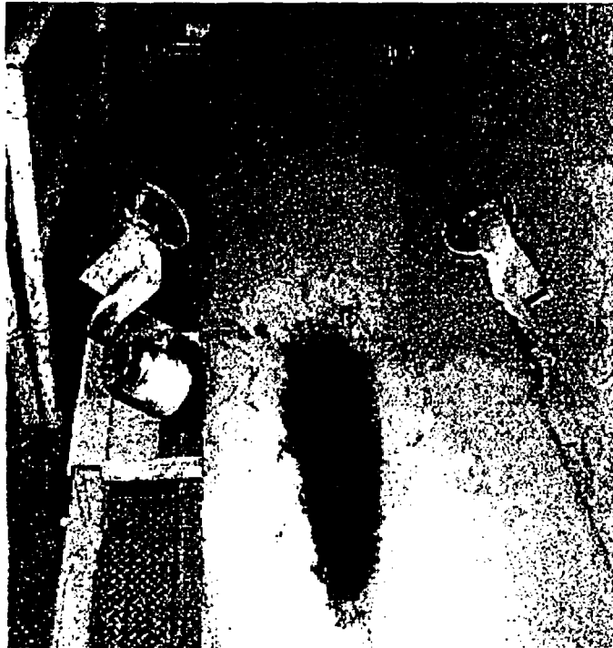
Figure 10. Station 25+20. Water collects on the conveyor behind the second bulkhead. There were at least three other puddles in the area. Water samples were collected by LBNL for analysis.
