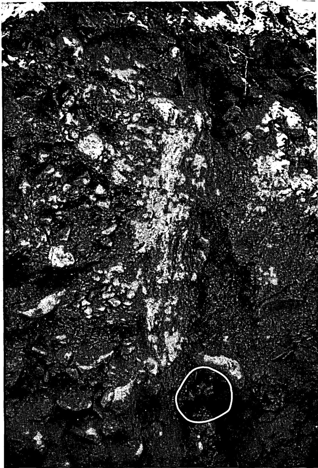
Figure 6.--Photograph of south wall of trench 1. Dark areas (circle near end of pick handle) are basalt ash. Sheared area to left is main fault zone. (Photo by W. J. Carr)
