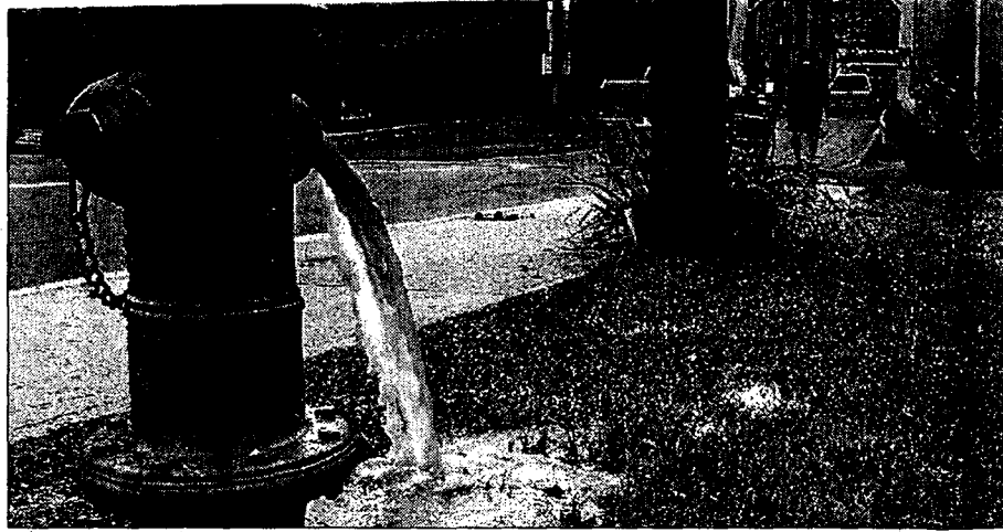
WITH UNDERGROUND pipes shaken in the earthquake, Milford, N.J., hydrant is open to air dirty water. Residents complained of tainted water.
