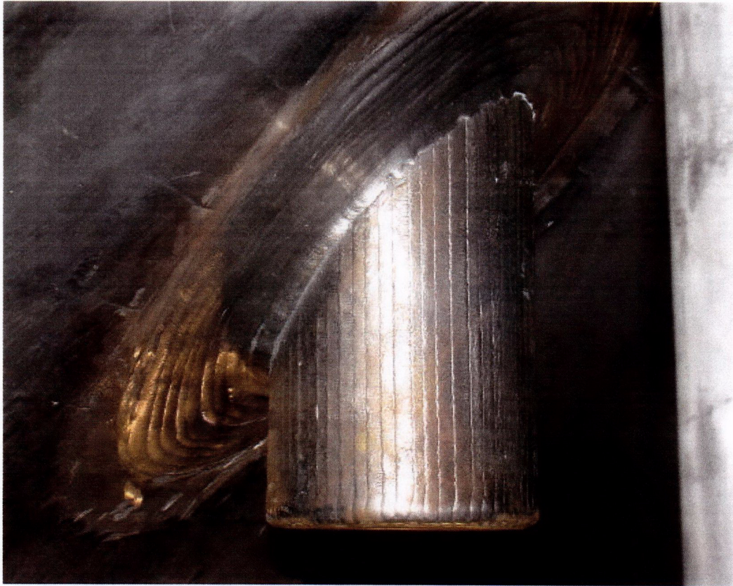
Figure 2: Weld Overlay Repair on another J-Groove Weld and Nozzle OD in the Jamesport Head Depicting the Rough As Welded Surface Condition over the J Groove Weld
