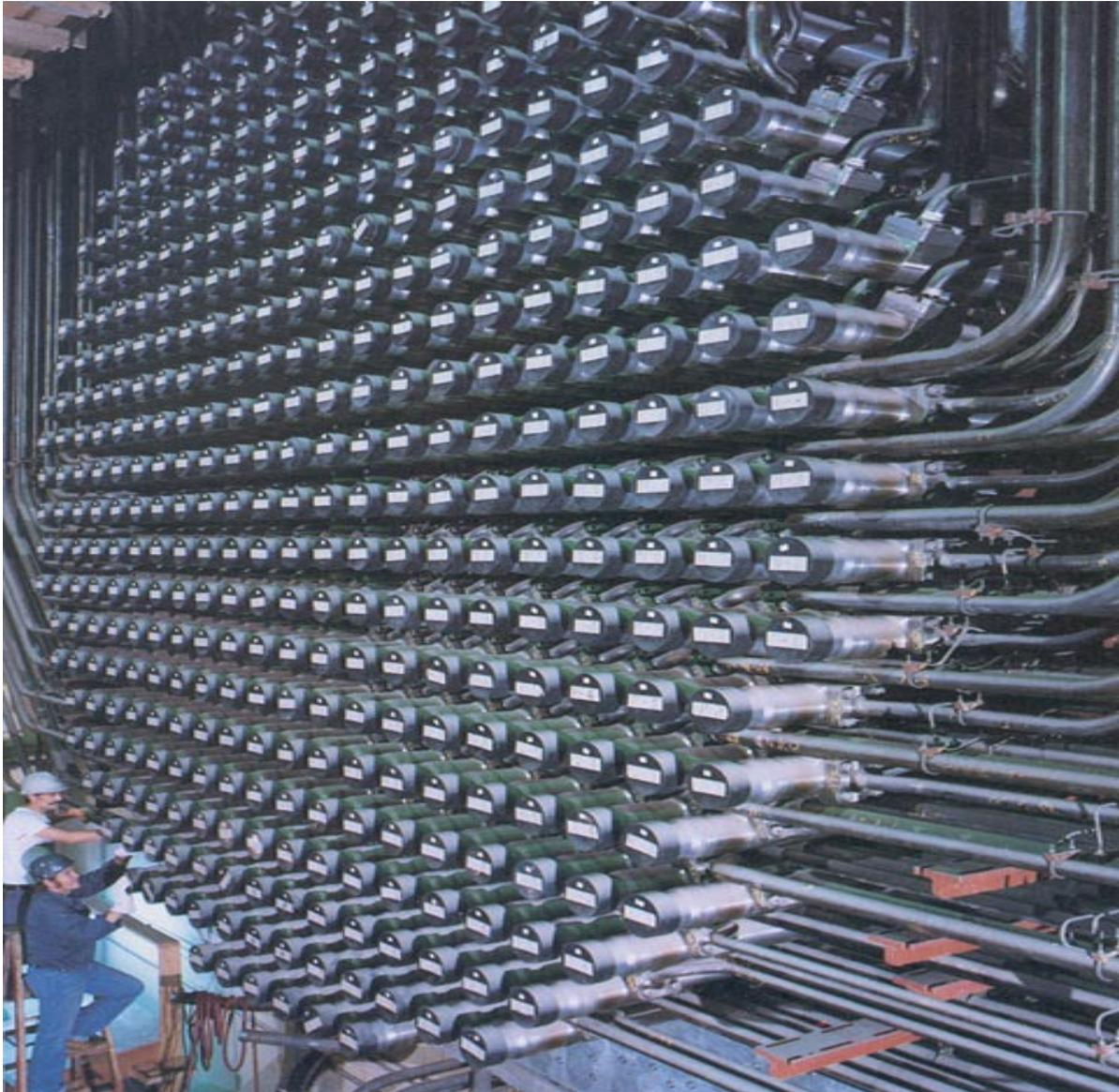
**Figure 1-3 The Face of a CANDU-6 Reactor as seen during Construction**
