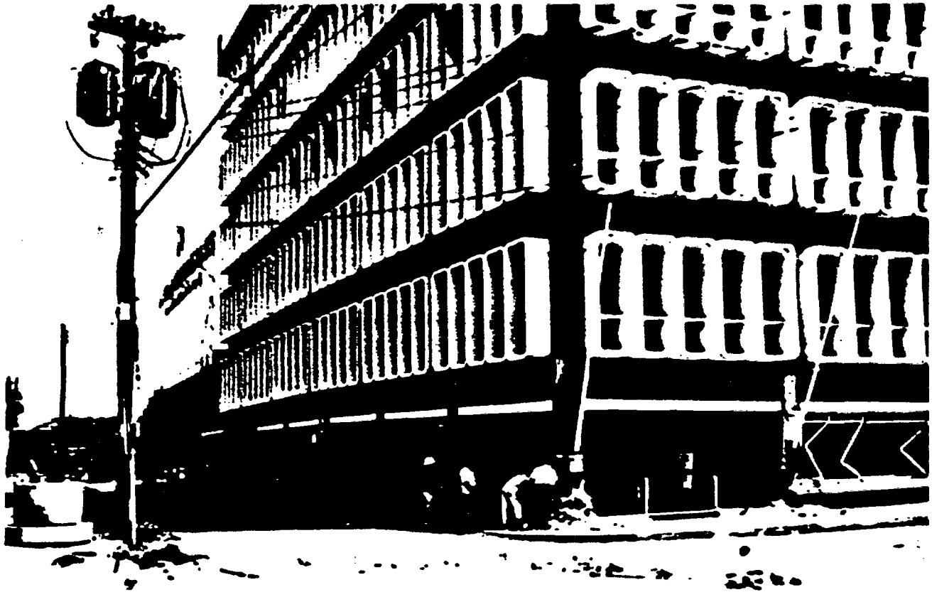
Fig. 4 — Philippine Bar Association building, Manila, 1968 earthquake.
