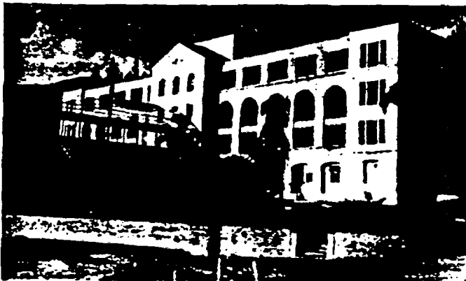
Fig. 5 — Two concrete shear-wall buildings of the Veterans Administration Hospital, San Fernando, California, 1971.
