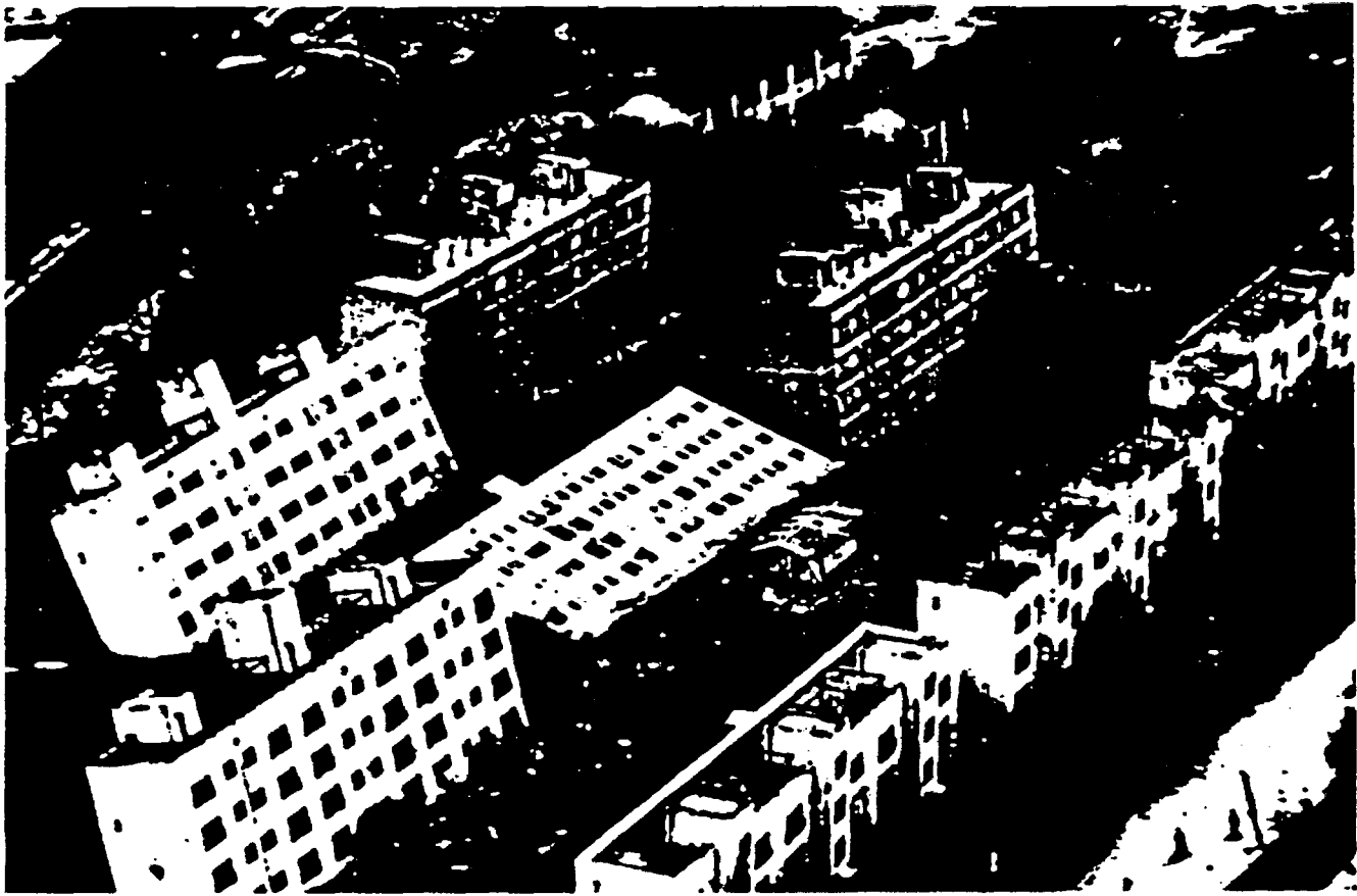
Fig. 12.— Ground failure due to liquefaction, Niigata, Japan, earthquake of June 16, 1964 (National Oceanic and Atmospheric Administration, U.S. Department of Commerce.)
