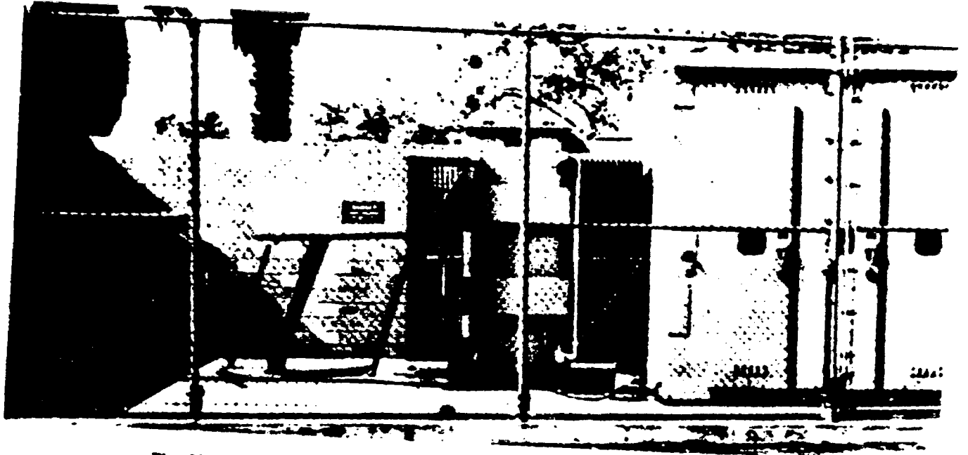
Fig. 22 — Olive View Hospital substation main transformer torn away from feeder cable.
