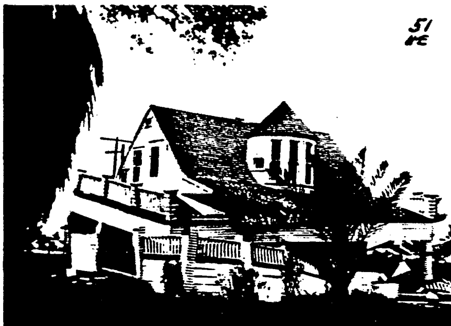
Fig. 9 — Wood-frame house, Long Beach California, 1933.
