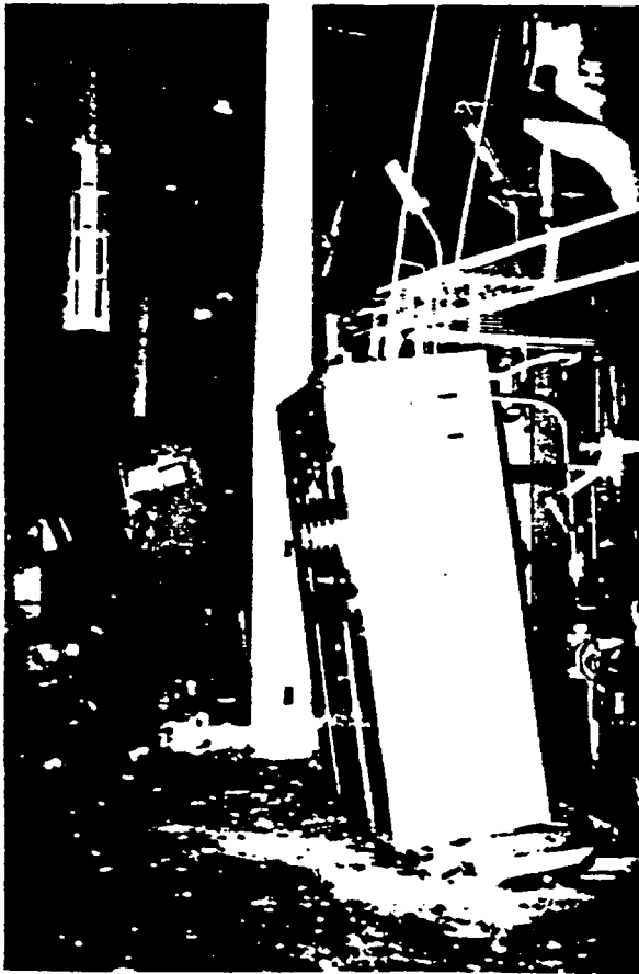
Fig. 20 — Motor control units in Olive View Hospital.
