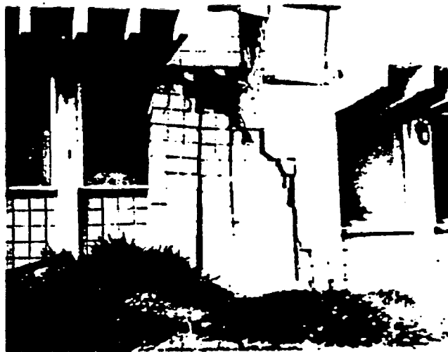
Fig. 8 — Stacked-bond laid, hollow concrete block wall with no reinforcing; San Fernando earthquake, 1971.
