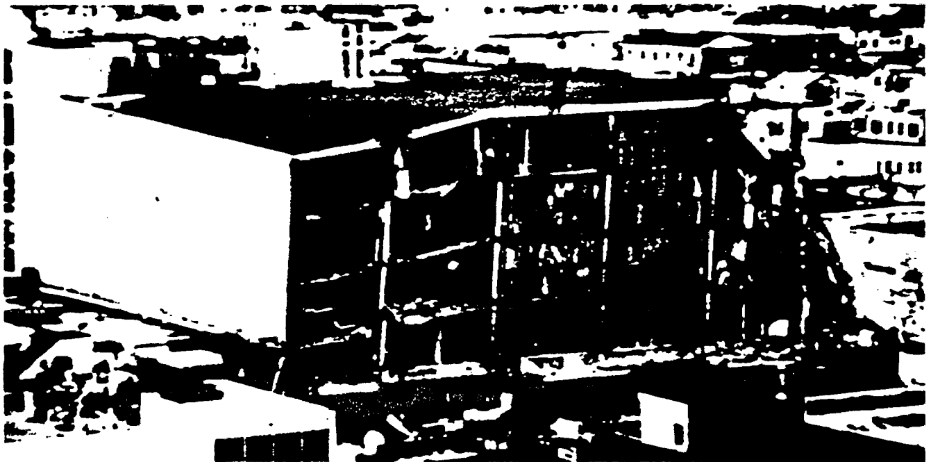
Fig. 7 — J. C. Penney building, Anchorage, Alaska, May 27, 1967 earthquake.
