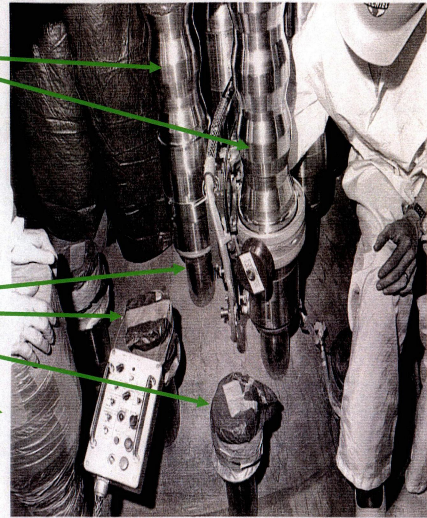
ANO-2 Head During Plant Construction
