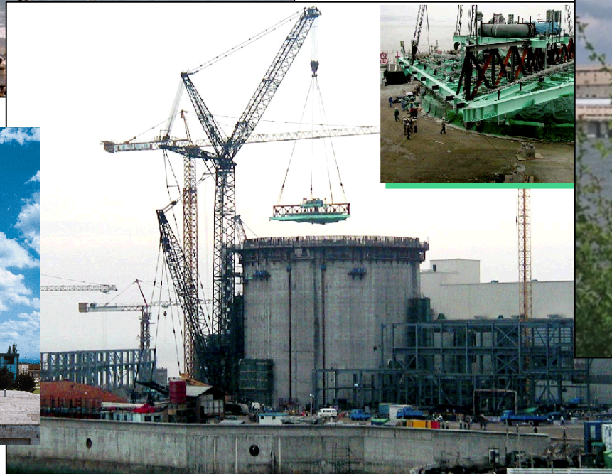
China – two units operating. Note open- top construction
