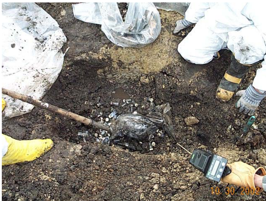
Figure 3-11: Use of a Photoionization Detector (PID) During Waste Removal
