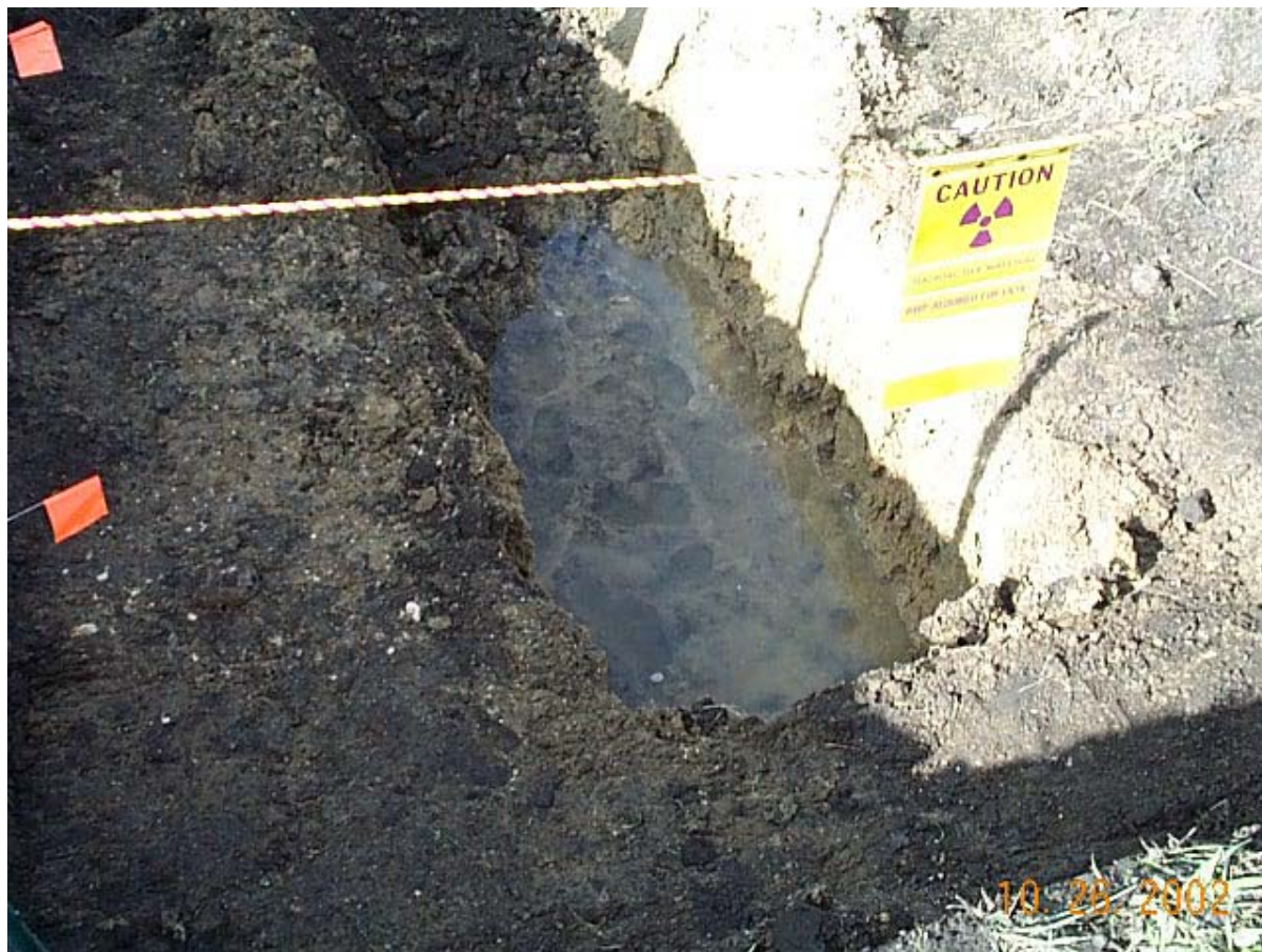
Figure 3-8: View of standing groundwater level in finished pit
