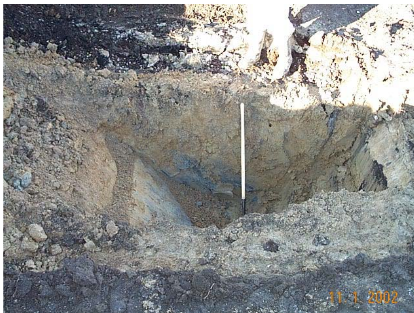
Figure 3-9: Pit 5 post-buffer soil removal. Discolored soil on north wall is seen to the left of shovel handle.
