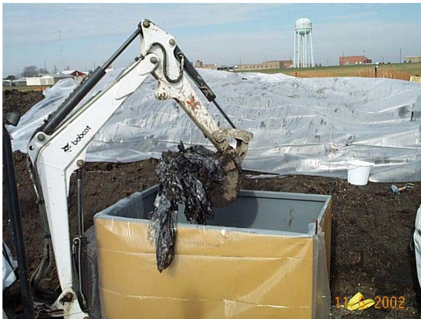
Figure 3-7: Loading of excavated wastes into B-25 box.
