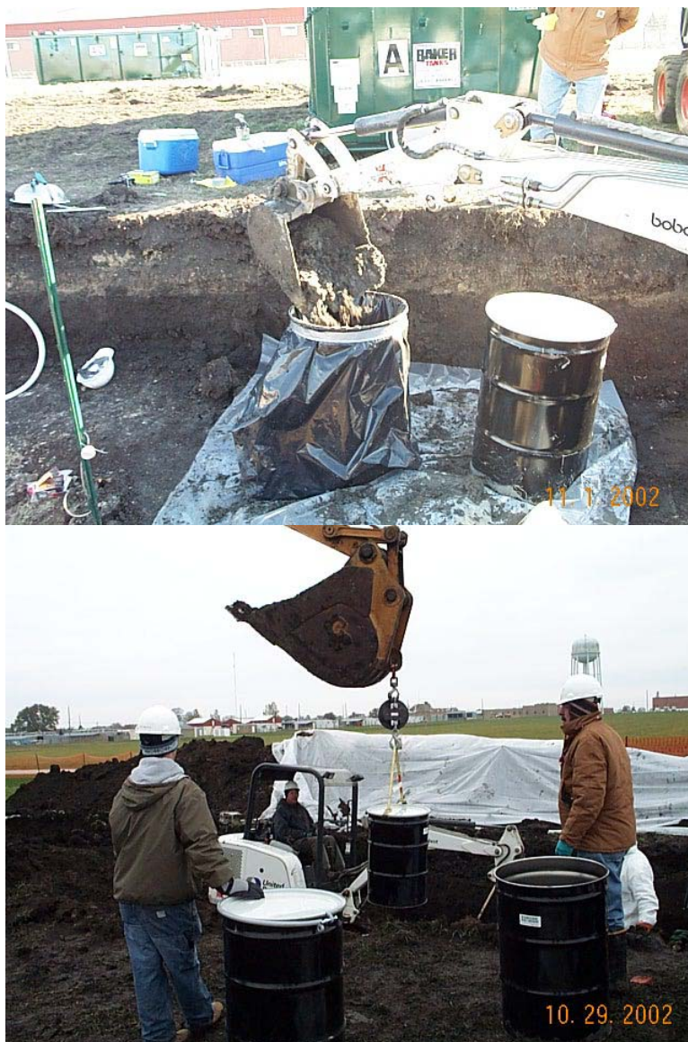
Figure 3-6: Photographs of drum loading and handling procedures during pit remediation
