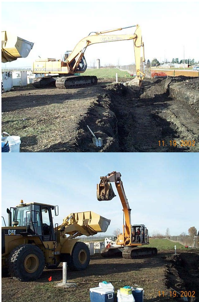
Figure 3-10: Buffer Soil Removal Process
