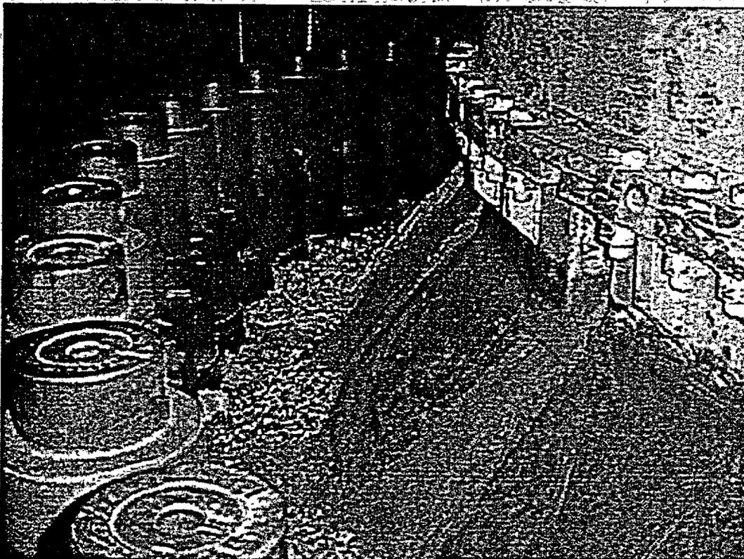
*Figure 4. Photograph taken at the 13<sup>th</sup> Refueling Outage (RFO 13) in 2000. The head bolts are seen at the left, and the service structure, housing the CRDM drive motors, the head insulation package and circulation fans, is shown at the right. The corrosion products flowed from a series of “mouse holes” – the square cutouts around the lower edge of the service structure skirt.*
