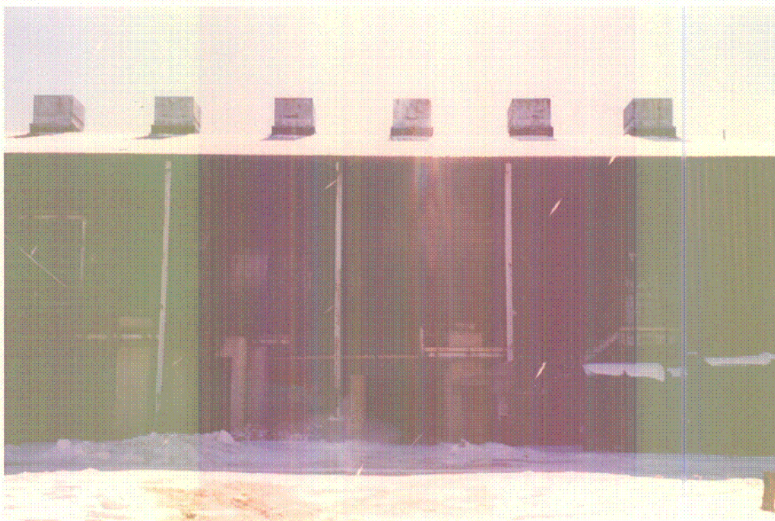
Dry Mill - Large 50 t/h Dryer Used Only by Asarco
