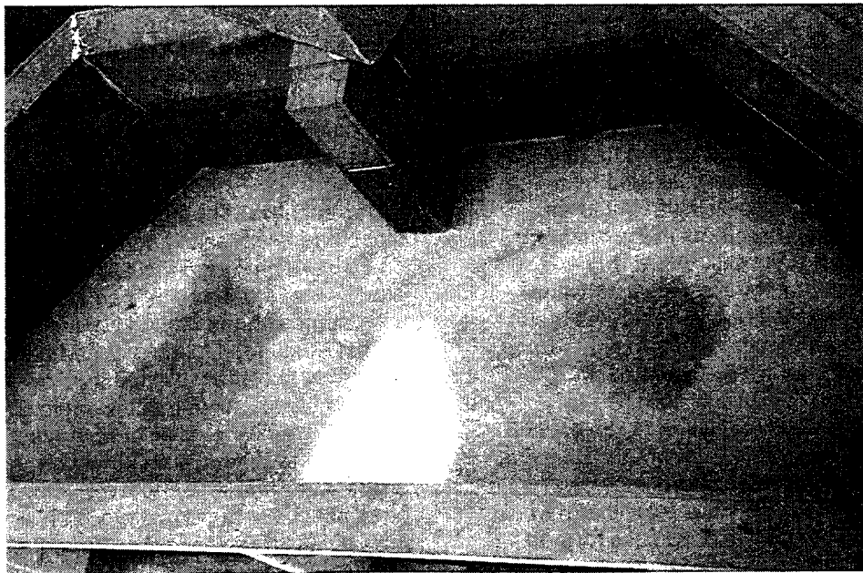
Figure 6-4 Debris Trapped in an Inner Compartment
