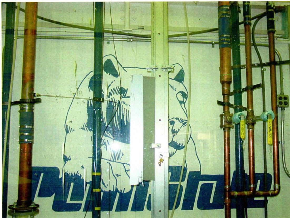
*Figure 4. Modified downcomer section: This design eliminates flow reversal to the steam separator and/or main condenser.*
