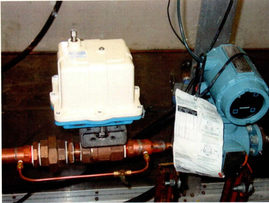
*Figure 5. Electric motor actuated valve and bypass valve.*
