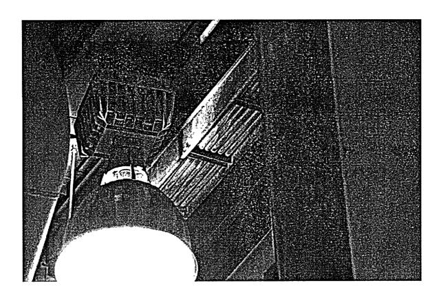
Further investigation revealed that the heat had indeed caused discolorations in the cable jackets, but this was only a surface effect is not a long-term potential problem.
