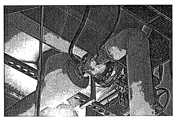
The photograph above was taken during the Oconee visual inspection walkdowns that led to the generation of the EPRI Adverse Localized Equipment Environment Guideline. This picture shows the power and control cables for an auxiliary steam (AS) system valve laying on top of an
