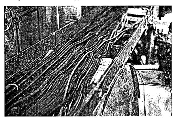
The visual signs that indicate aging degradation of cables in the tray are the way the cables "droop" between the cable tray lattice supports and many of the cable jackets look "dry" and have surface cracks.
