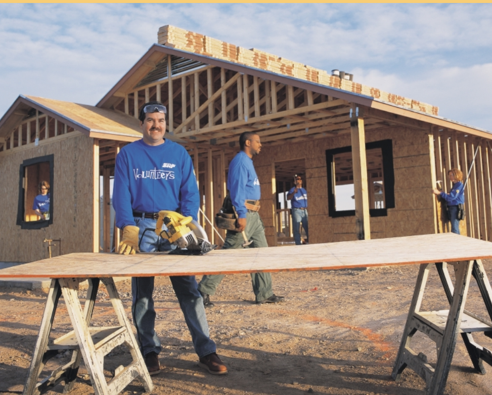
This year, SRP volunteers helped to build their fifth Habitat for Humanity home in Phoenix, providing a permanent residence for another family in need. Michael Krause, an SRP operations manager, worked with more than 100 SRP volunteers and others to make the home complete.
