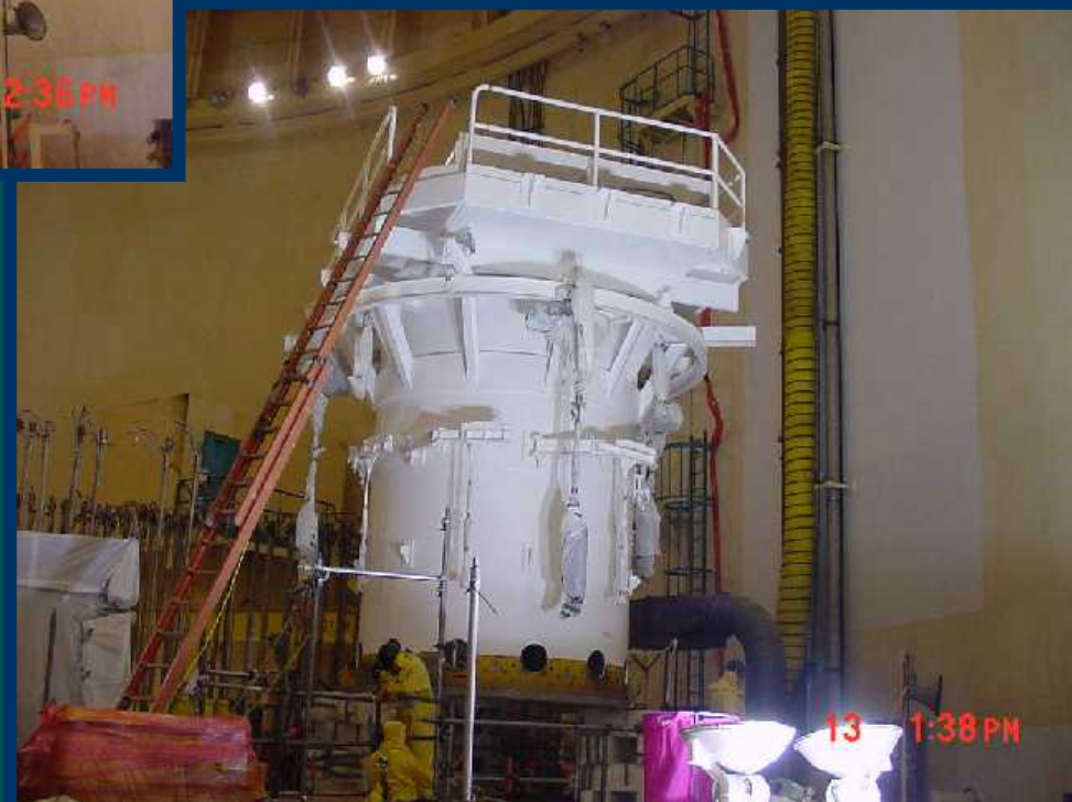
After Sponge Jet-Blasting and Painting
