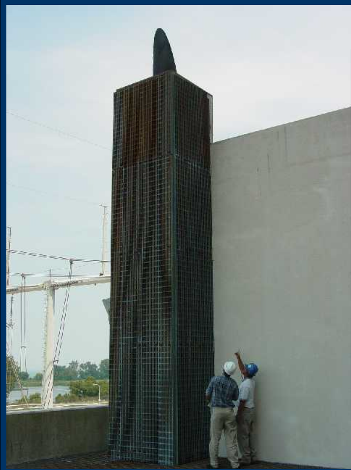
Emergency Diesel Generator Base Plate for Missile Shield
