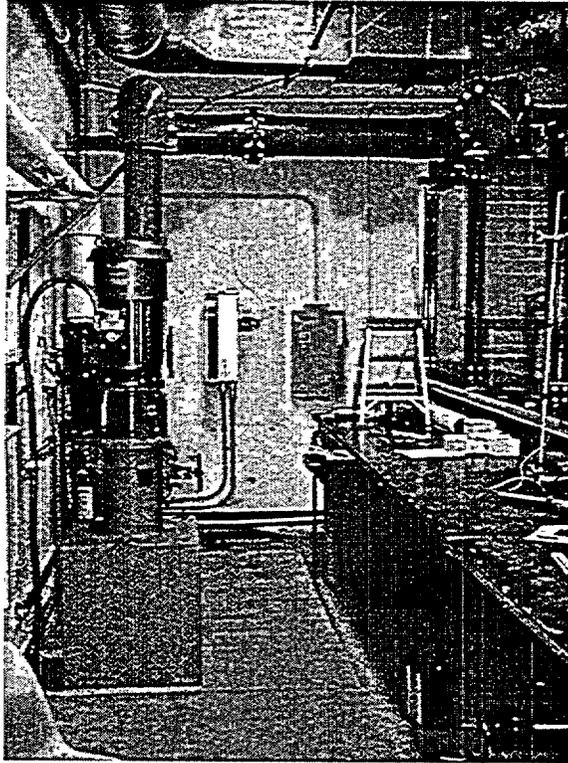
**Figure A.15 Large Flume Supply Pump and Overhead Piping**
