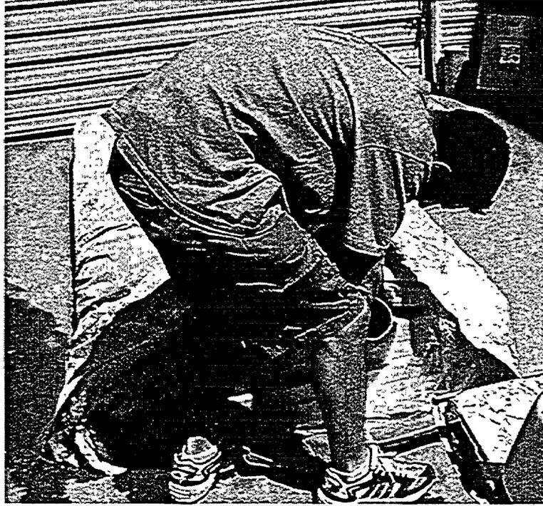
**Figure 3.2a Thermal-Wrap Fiberglass Insulation in Bulk Form**
