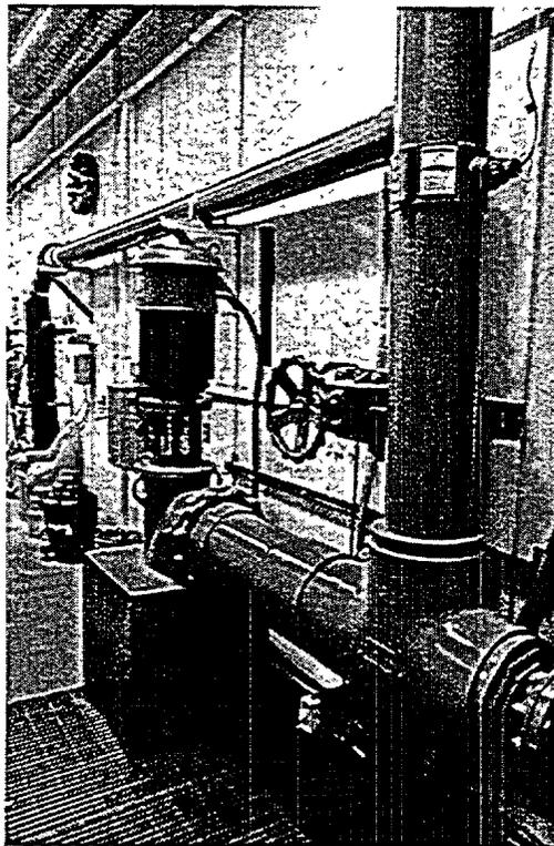
**Figure A.16 Large Flume Supply Pump and In-Line Flow Meter**
