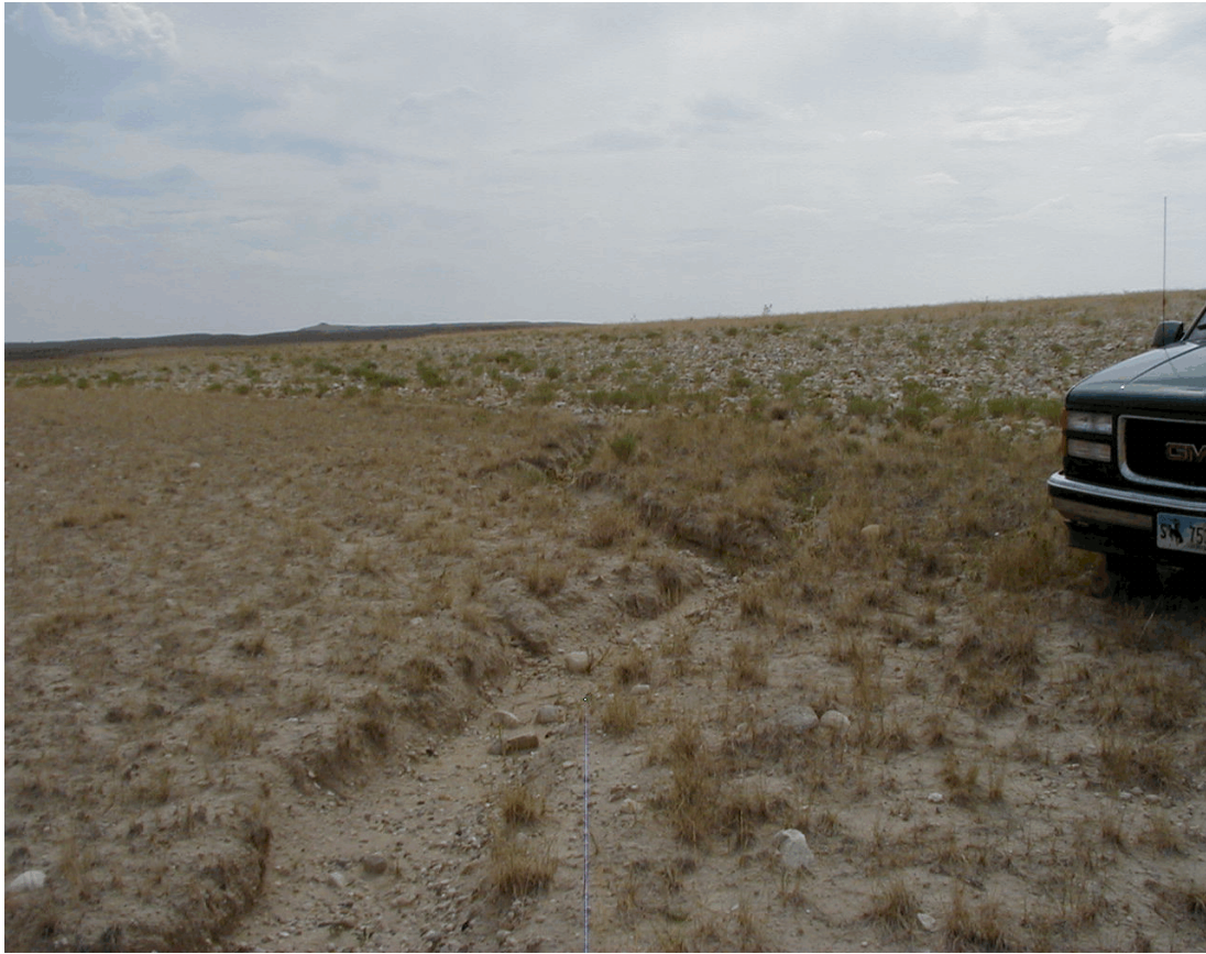
Gullying at edge of ANC No. 2 Tailings Impoundment
