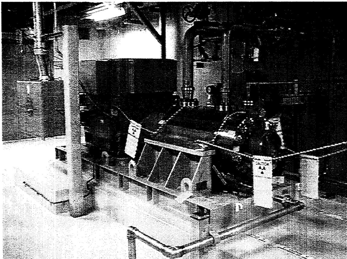
**Figure 5. Photograph of Normal Charge Pump (CAM model), Plant Installation (Callaway Nuclear)**
