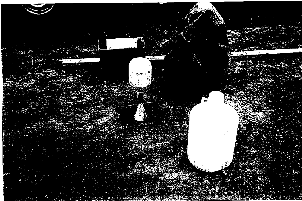
Figure 7. Typical sand cone test.
