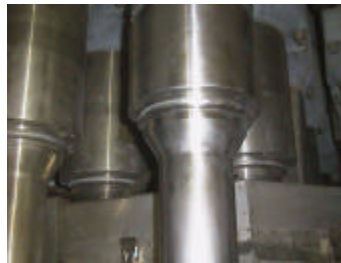
Figure 12 - CRDMP No. 75 L-15 Conoseal/CRDM Column (After Cleaning)
