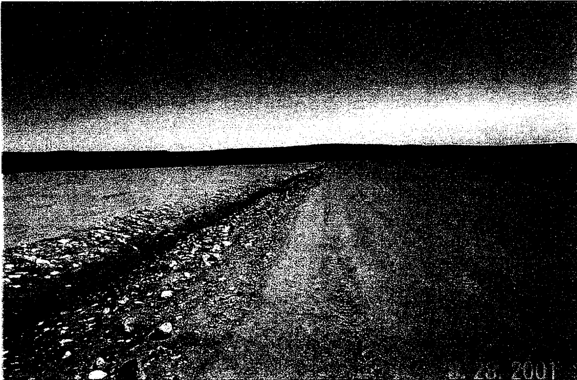
Photo A.13.1 Looking north down south low-flow channel, with accumulation of windblown soil in channel. (Aug 2001)
