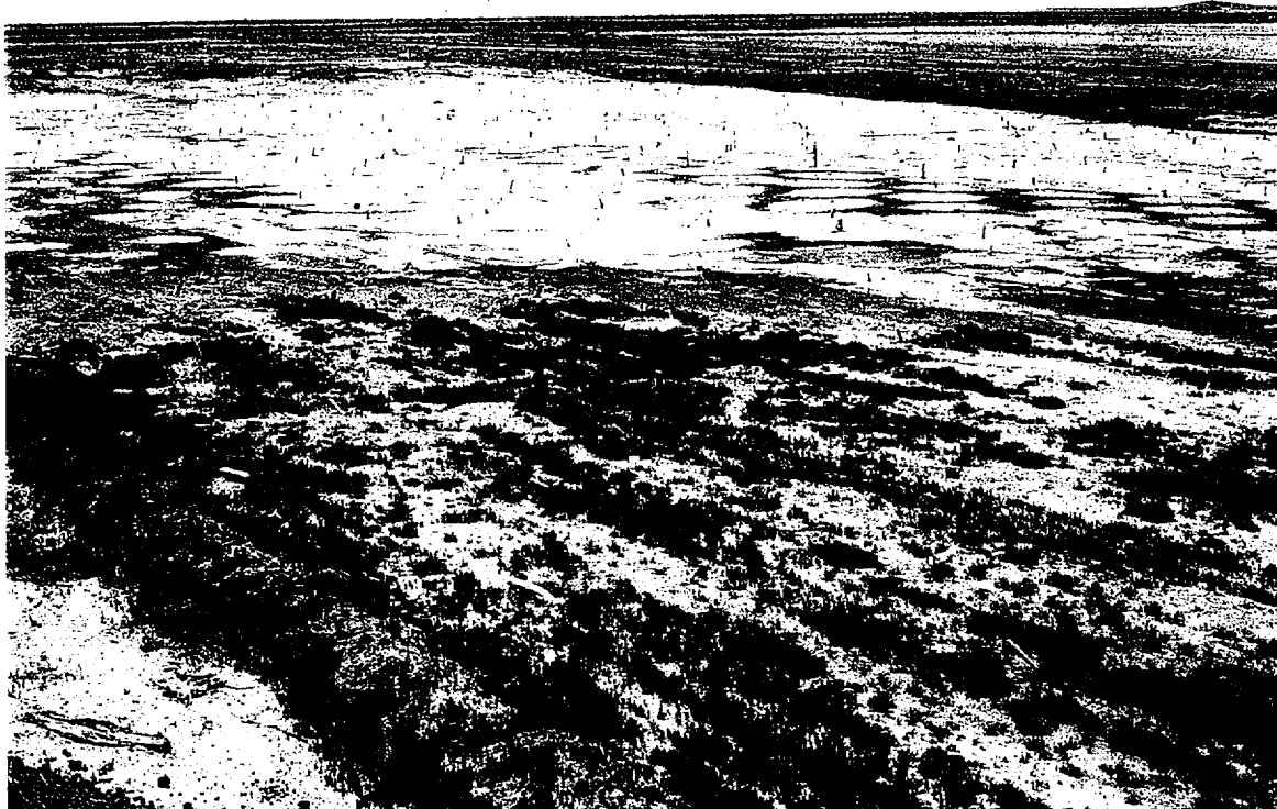
Photo A.2.2 Wick area, with end of vertical band drains (wicks) showing above random fill surface. (Jun 1989)
