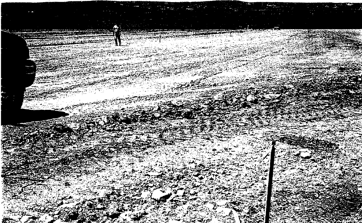
Photo A.9.2 Looking northwest across fill placement area after 2000-2001 construction. Final grading of topsoil is taking place. The first lift of rock in the south low-flow channel is in the foreground. (Jun 2001)
