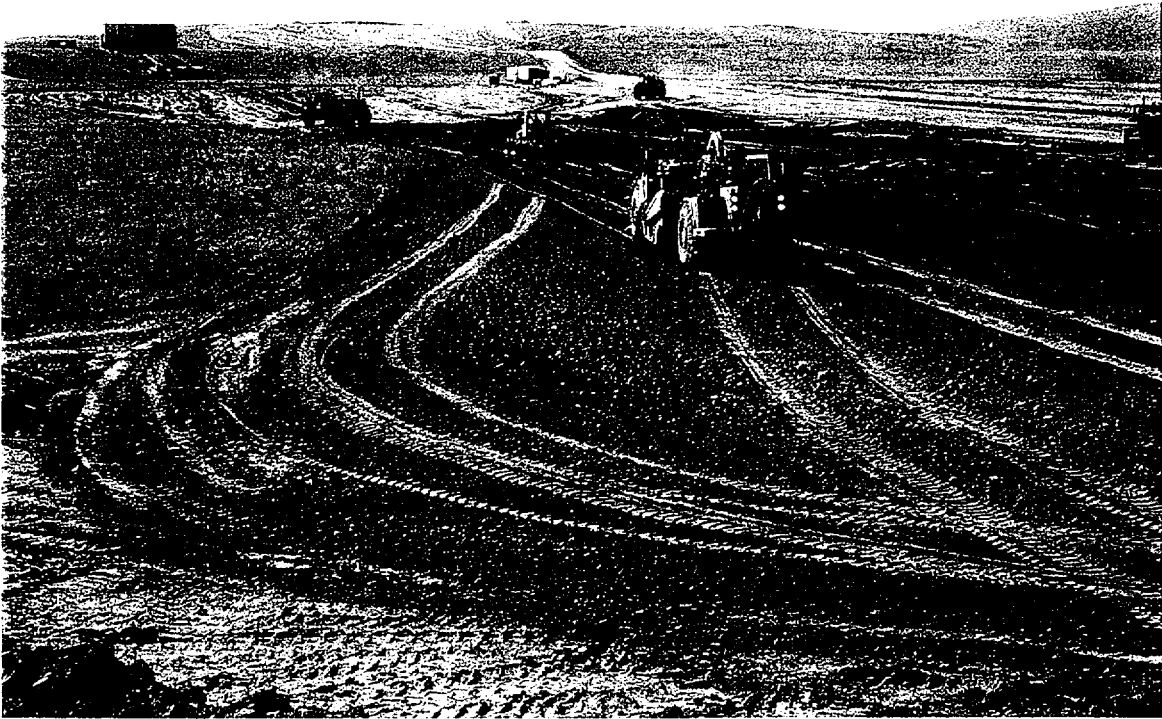
Photo A.6.1 Radon barrier placement during 2000-2001 construction. Water storage tanks are at left and the Middle Dump borrow area is in the distance. (Apr 2001)
