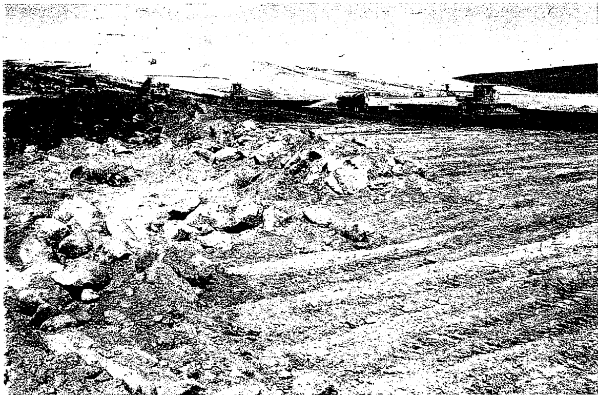
Photo A.3.2 Random fill placement (at left) and radon barrier placement (at right) during 1989 construction. The Middle Dump borrow area is in the distant center of the photo. (Jul 1989)
