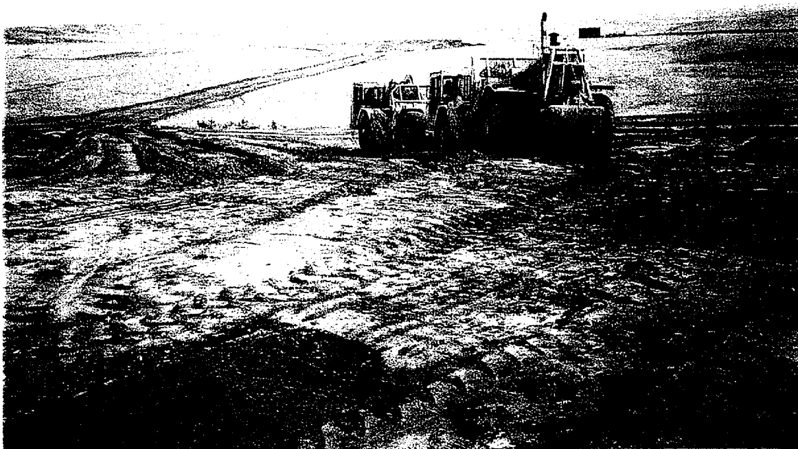
Photo A.6.2 Looking toward fill placement area from Middle Dump borrow area during 2000-2001 construction. Typical Middle Dump materials are in the foreground. (Nov. 2000)
