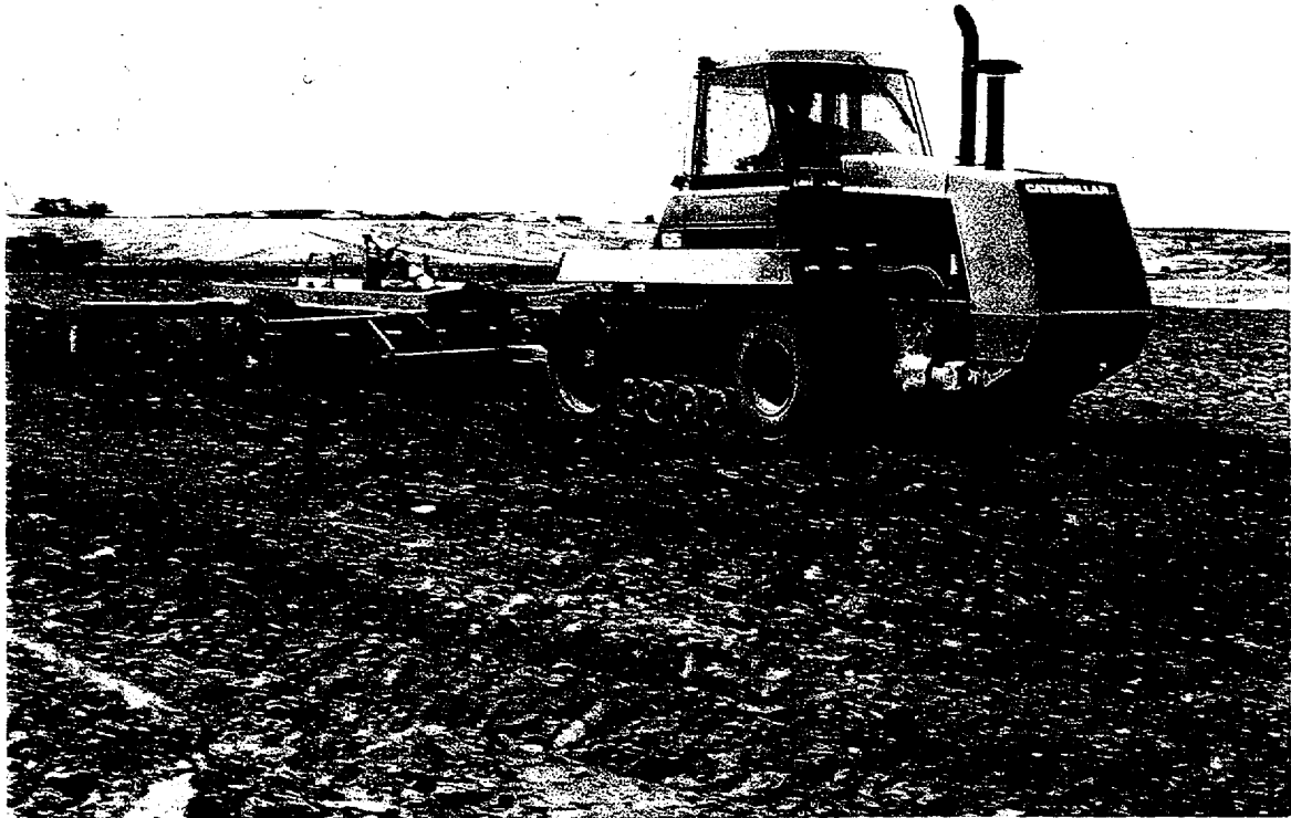
Photo A.4.1 Moisture conditioning of radon barrier material during 1989 construction.
