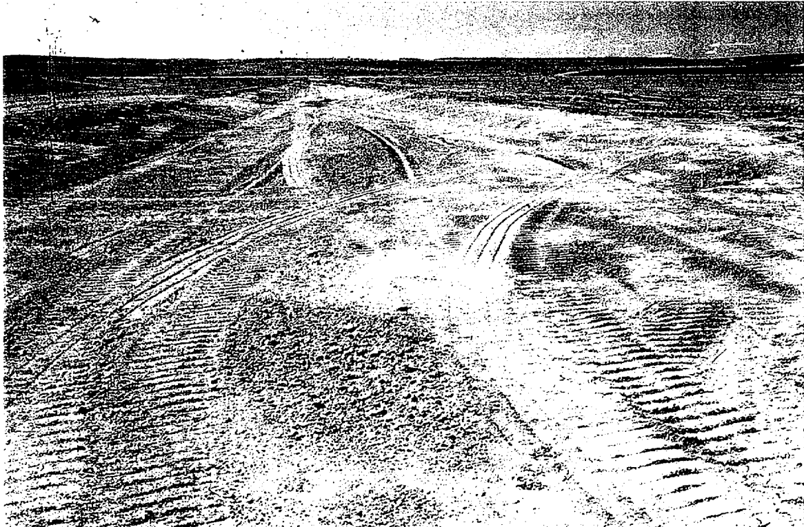
Photo A.5.1 Looking southward up the south low-flow channel from junction with west low-flow channel. Channels have been shaped and topsoil placed to edge of channel prior to rock placement. One of the cover soil stockpiles is on the right side of the photo. (Sep 1989)
