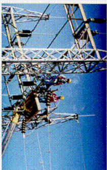
(L) CIPCO employees from the Creston crew replace lightning arresters at the Summit Lake South substation. (R) CIPCO line crew work with linemen from SWISCO to install temporary service at the Carbon Substation to ensure customers will not lose service during installation of a new transformer.
