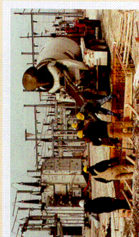
A new natural gas pipeline was installed to the Summit Lake Generating Plant to supply additional fuel to the combustion turbines.
