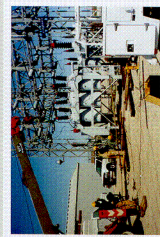
Improvements are made to the system by installing gas breakers to replace obsolete oil circuit breakers at Grand Mound Substation.
