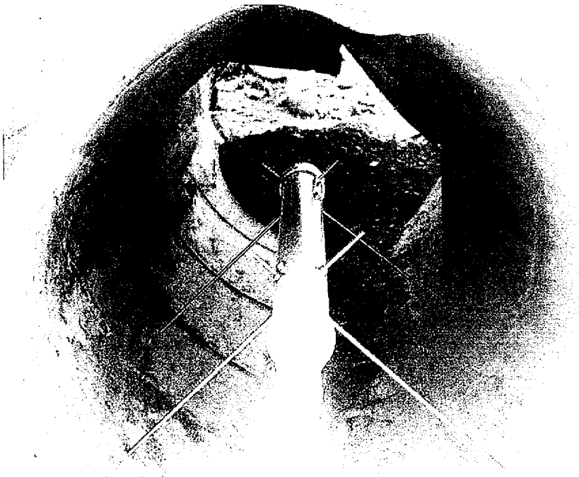
Photograph 4.2a – Cross-Over Line Between Intake Tunnel to Spray Pond
