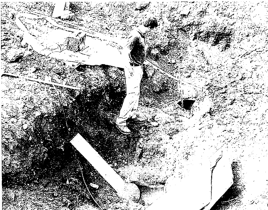
Photograph 4.5b – Center Yard Drain Pipe, Excavated Behind Garage (foreground)
