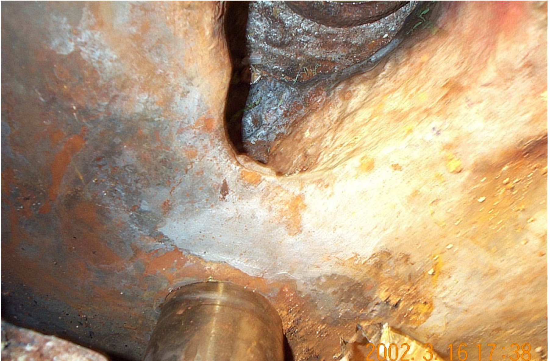
Nozzle 3 with insulation removed and shielding installed 03-16-02
