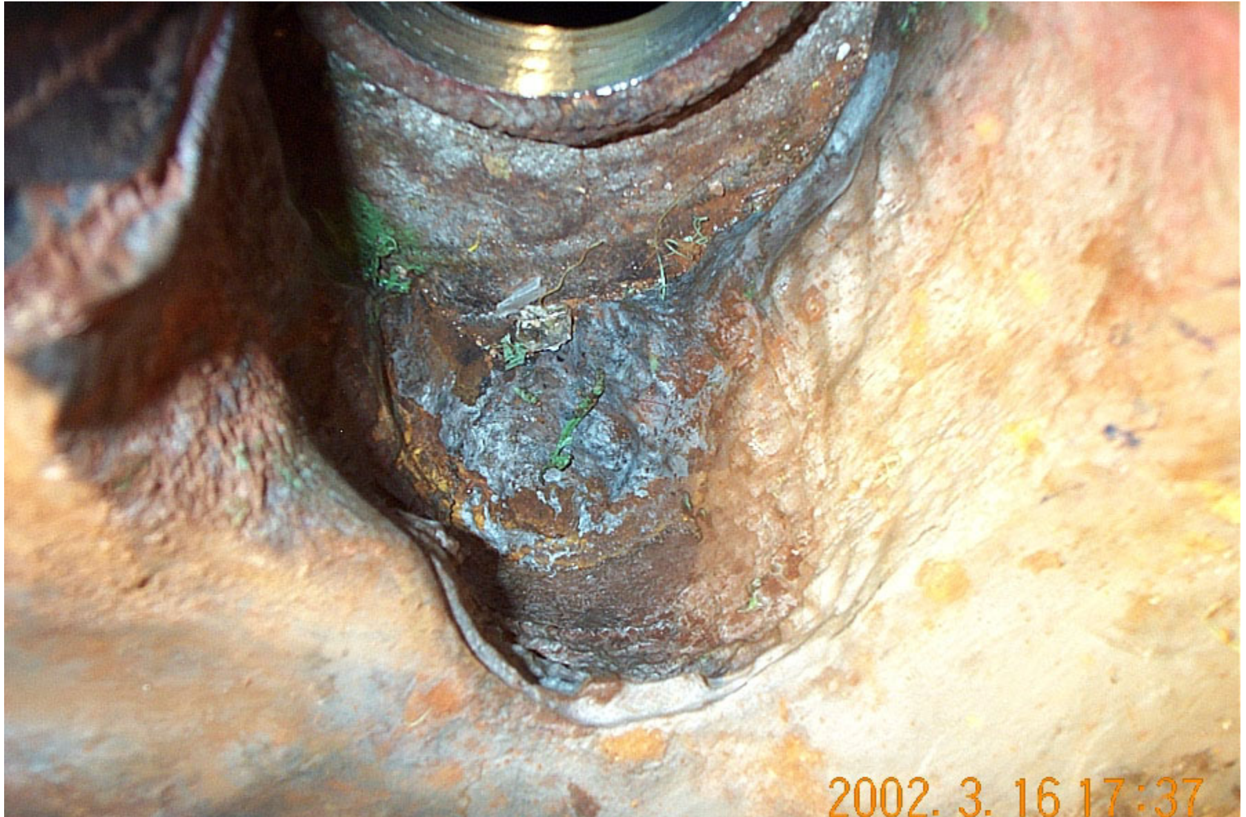
Nozzle 3 with insulation removed and shielding installed 03-16-02
