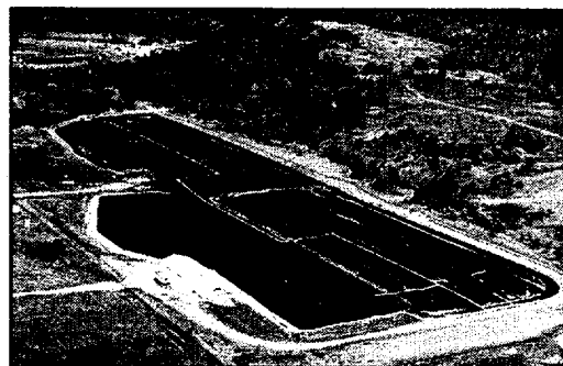
A polymer cover and subsurface clay barrier have controlled water infiltration into the SDA trenches.
