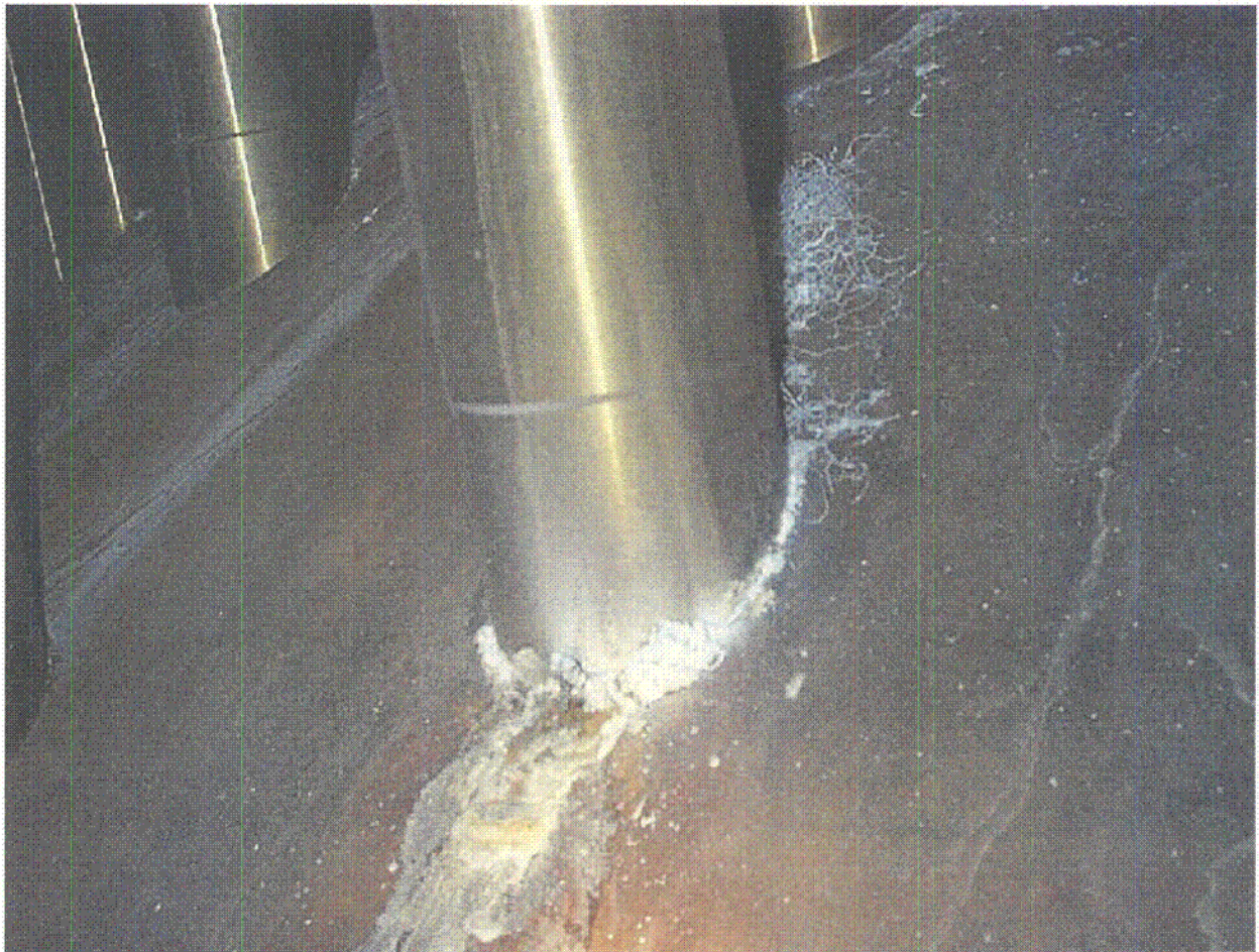
Figure 18. CRDM Nozzle Leakage Observed at Oconee 3
