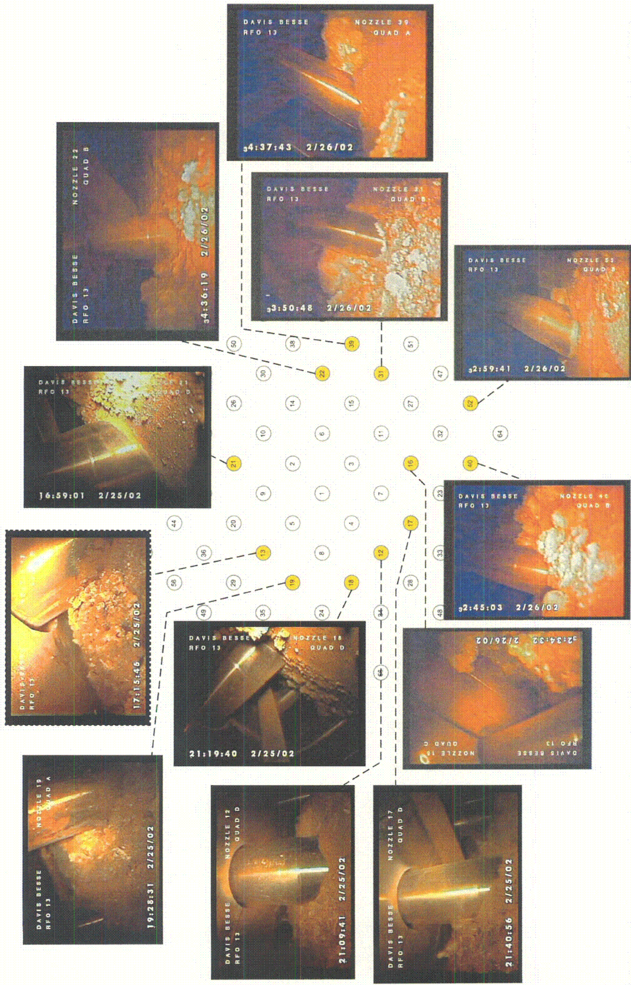
Figure 24. Boric Acid Deposits on Top of Head at Start of 13 RFO
