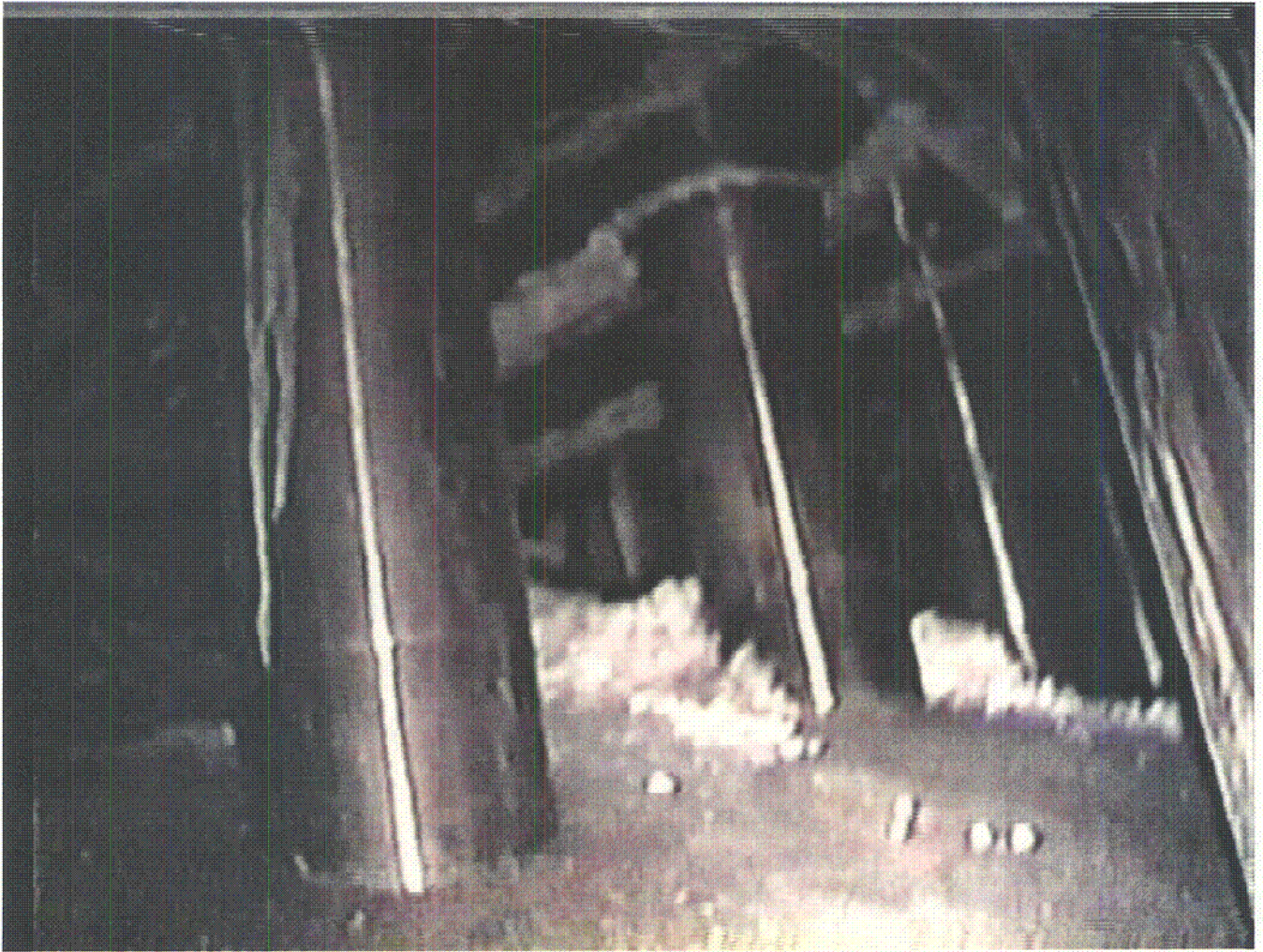
Figure 33. North Side of Reactor Vessel Head (10RFO)
