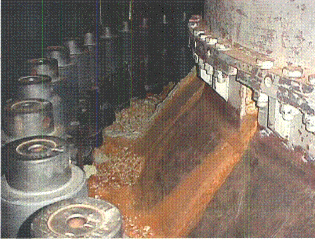
Figure 4. Boric Acid and Iron Oxide on Vessel Flange at 12RFO
