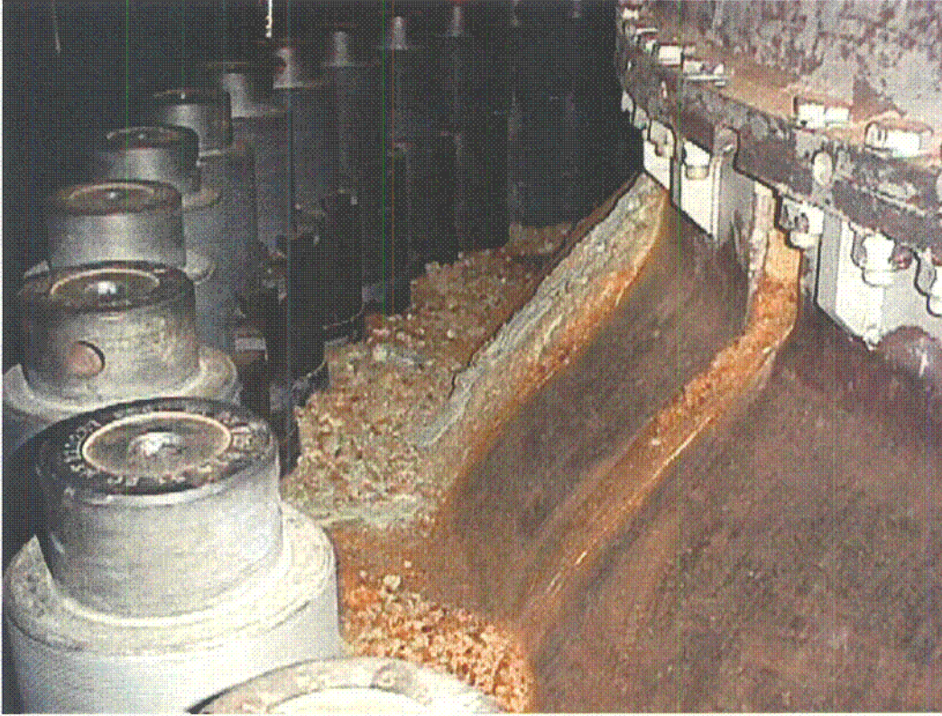
Figure 36. Red Rusty Boric Acid Deposits on Vessel Flange (12RFO)
