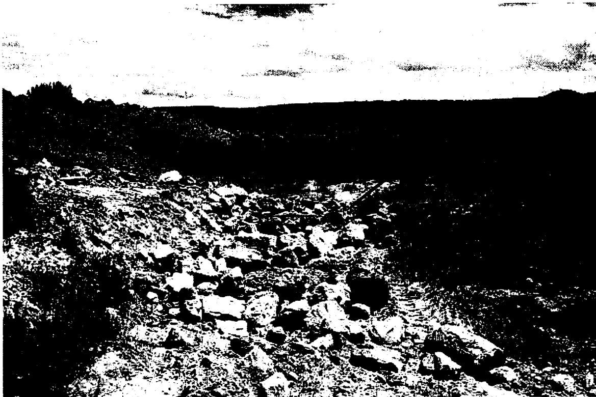
PL-3. Riprap Armor in Ditch Number 1 at Fence Line
