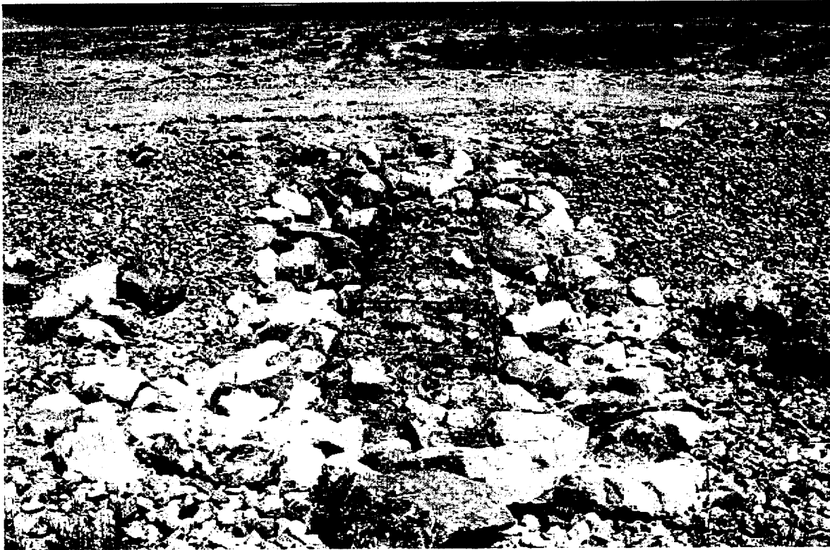
PL-1. Riprap Armoring for Ditch Number 1 Gabion
