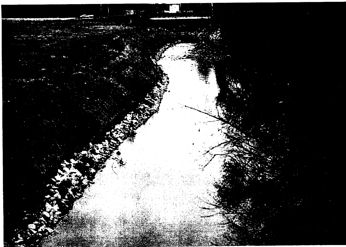
PL-2. Stabilized Western Bank Of Chartiers Creek at Area C
