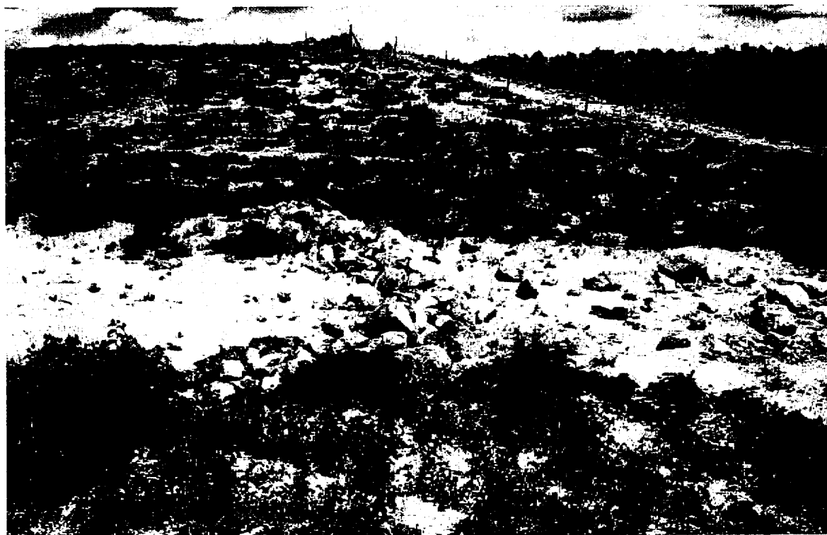
PL-4. Erosion Protection Near the Property Line Along Swale Number 1
