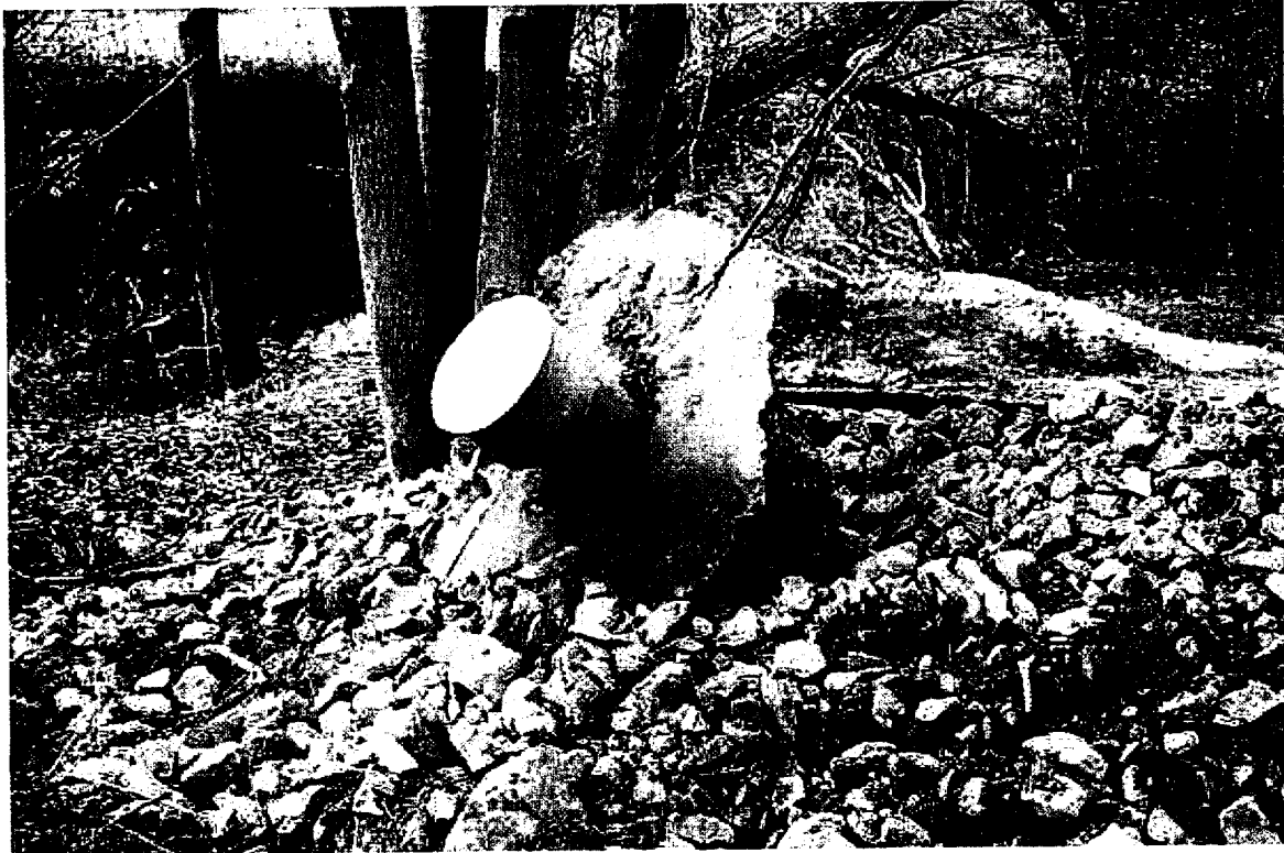
PL-1. Displaced Cap of Destroyed Monitor Well 0406
