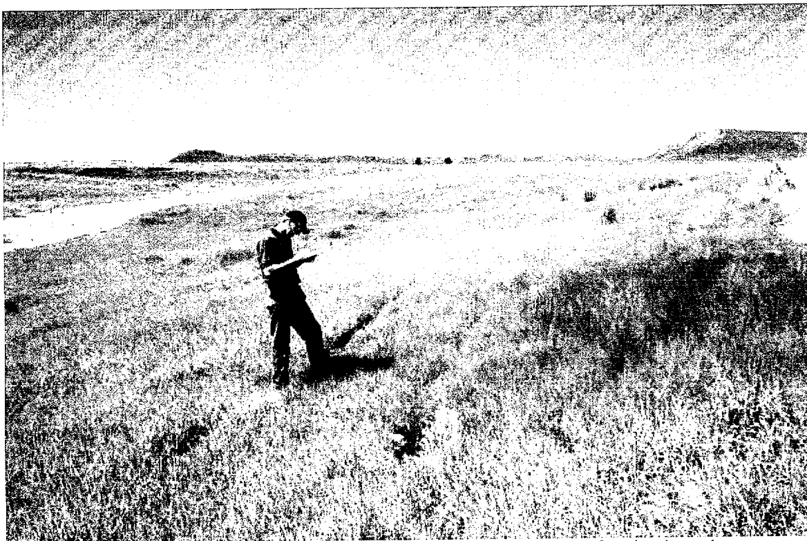
EDG 6/2001. PL-2. Tire tracks on top slope near west end of embankment.
