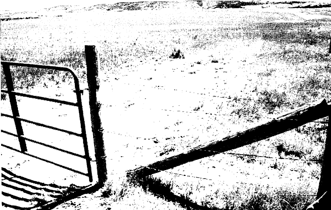
EDG 6/2001. PL-1. Dislocated horizontal member of "H" brace at entrance gate.
