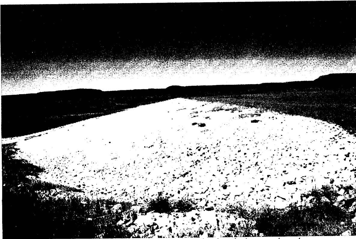
EDG 6/2001. PL-3. Embankment face showing plant encroachment.
