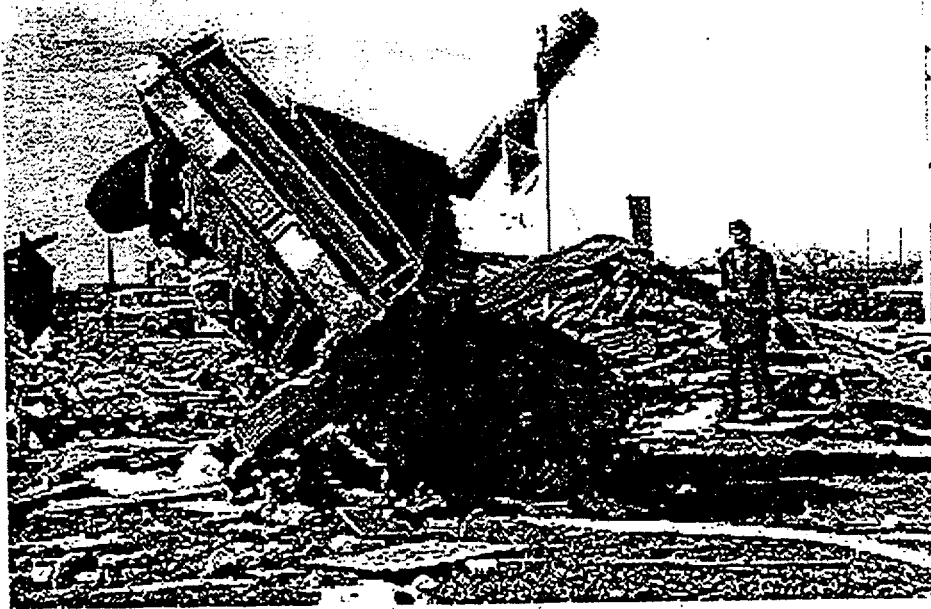
FIGURE 2.20 AN AUTOMOBILE THAT WAS SLAMMED AGAINST A STEEL POLE IN BOSSIER CITY, LOUISIANA (FS, 1978)
