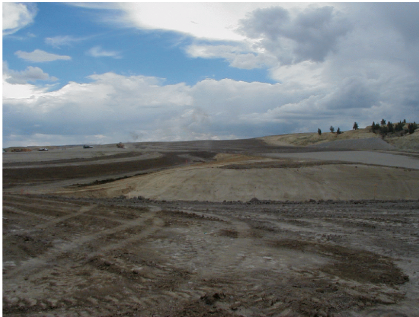
Pathfinder Upper Channel North West
