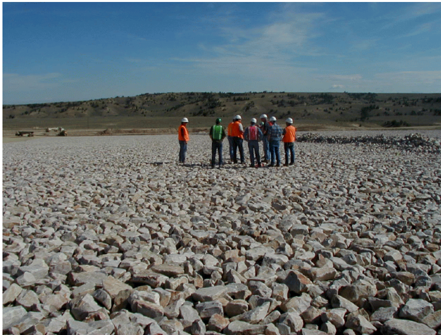
Twelve Inch Rock Placement on UMETCO Above Grade Tailings Impoundment
