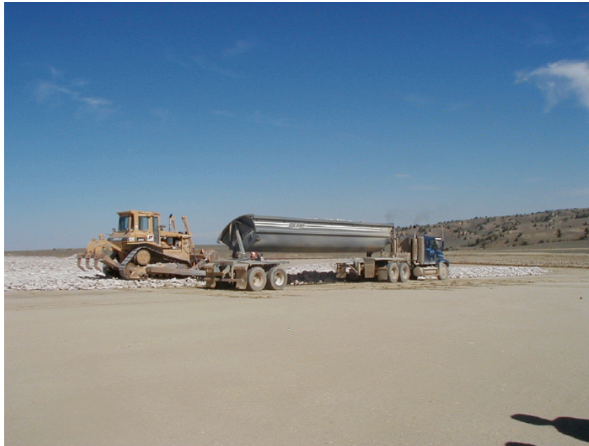
Dumping and Placement of Twelve Inch Rock
