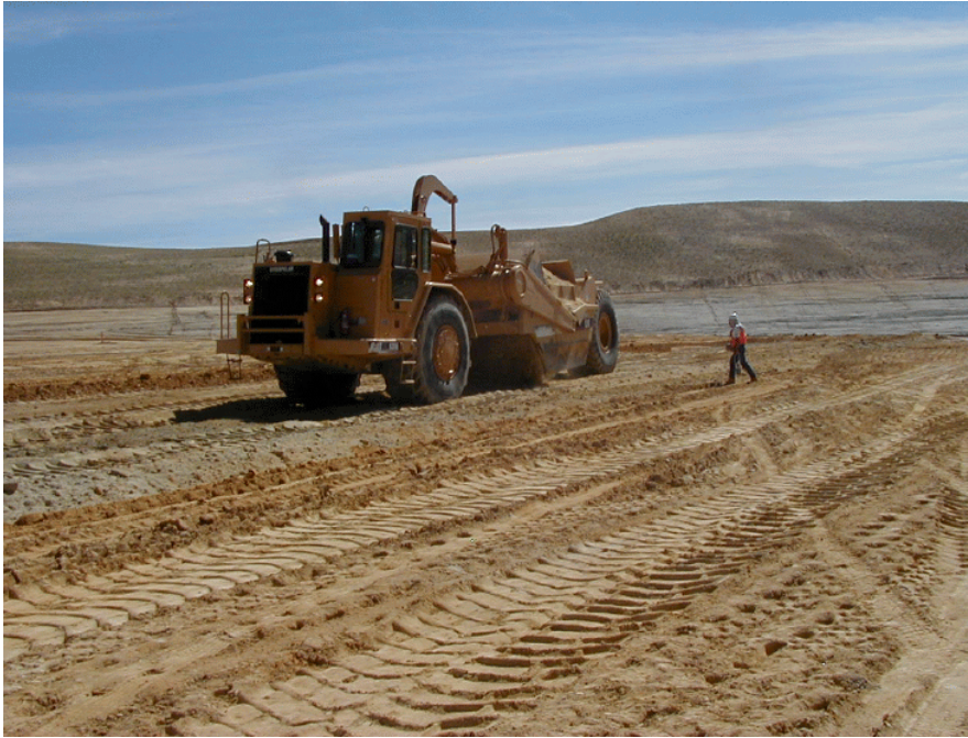
Placement of Cover Material on C-18 Pit
