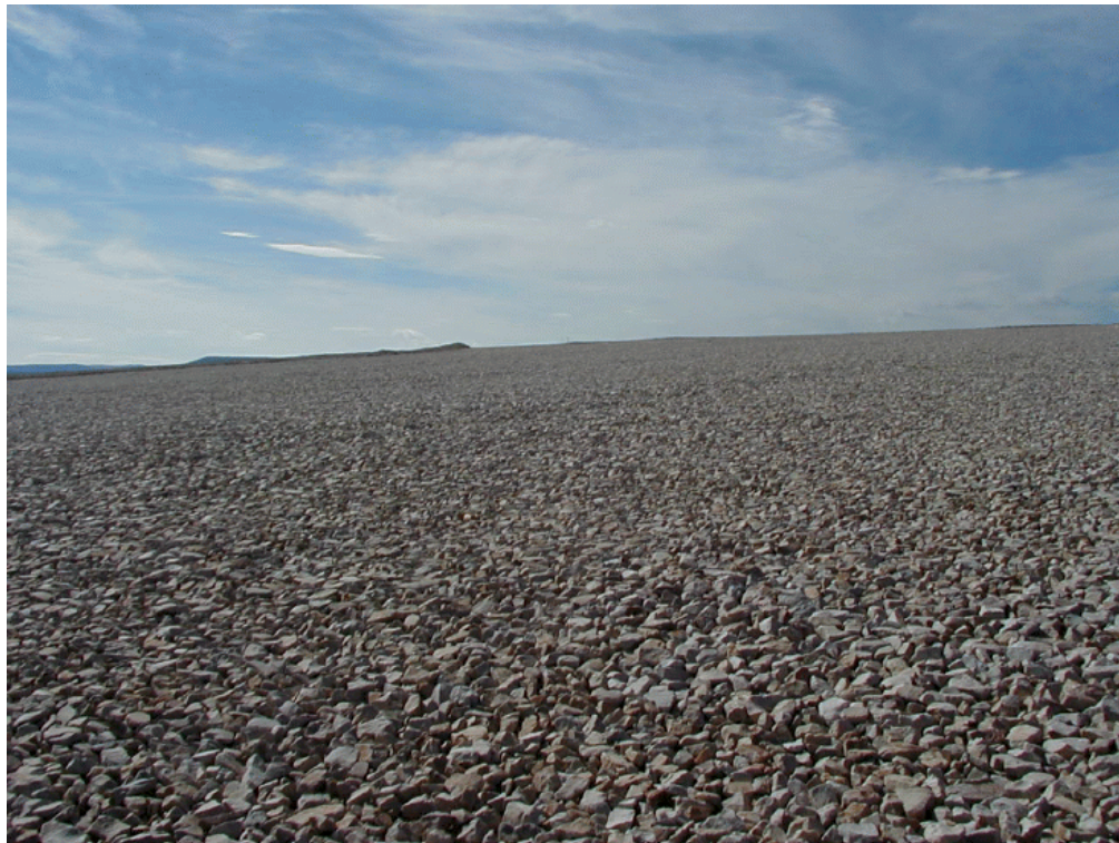
Six inch rock placement on UMETCO Above Grade Tailings Impoundment
