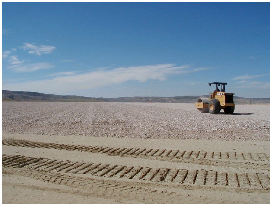
Compaction of Three inch Rock on the Top of the Above Grade Tailings Impoundment
